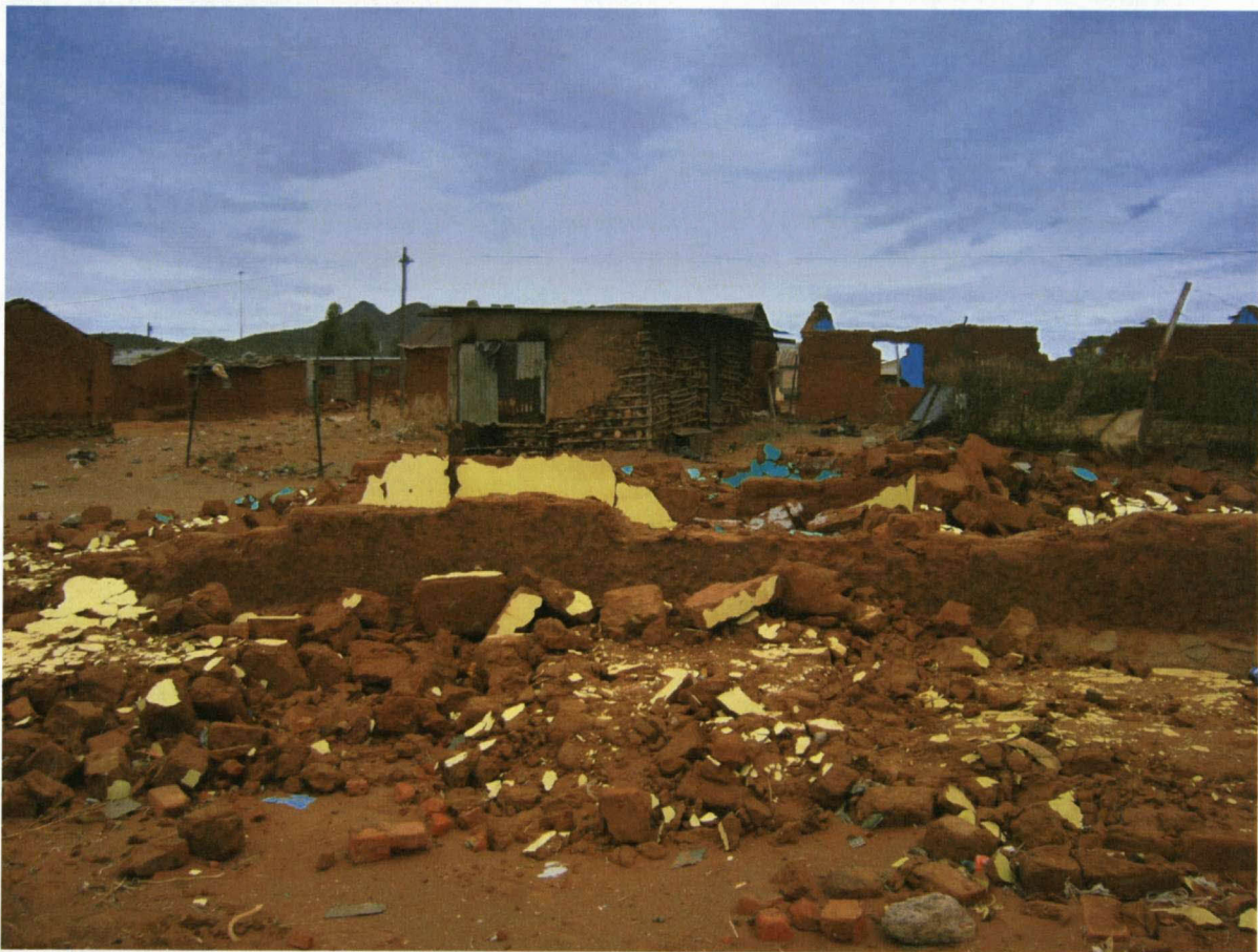
Figure 4.11: A demolished vernacular home in Luxolweni, 2007
