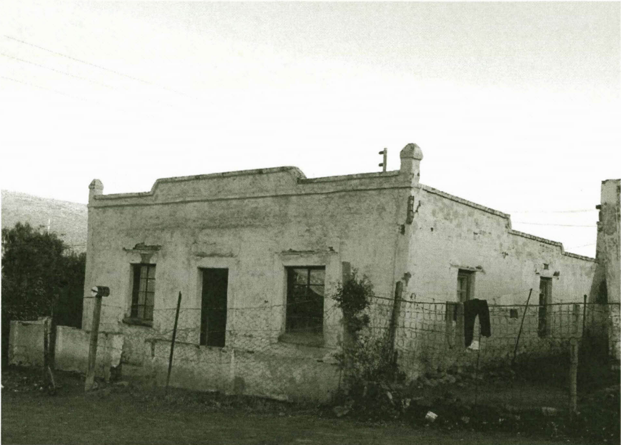
Figure 3.6: Example of flat-roofed or brakdak houses found within uMasizakhe
