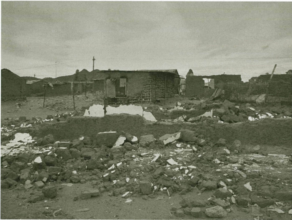
Figure 4.11: A demolished vernacular home in Luxolweni, 2007
