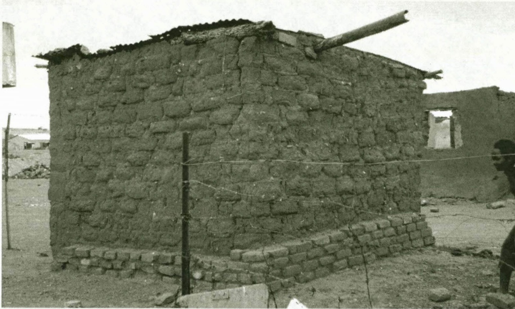
Figure 4.15: Adobe blocks laid on a plinth of sundried bricks as well as various materials used to support corrugated iron roof
