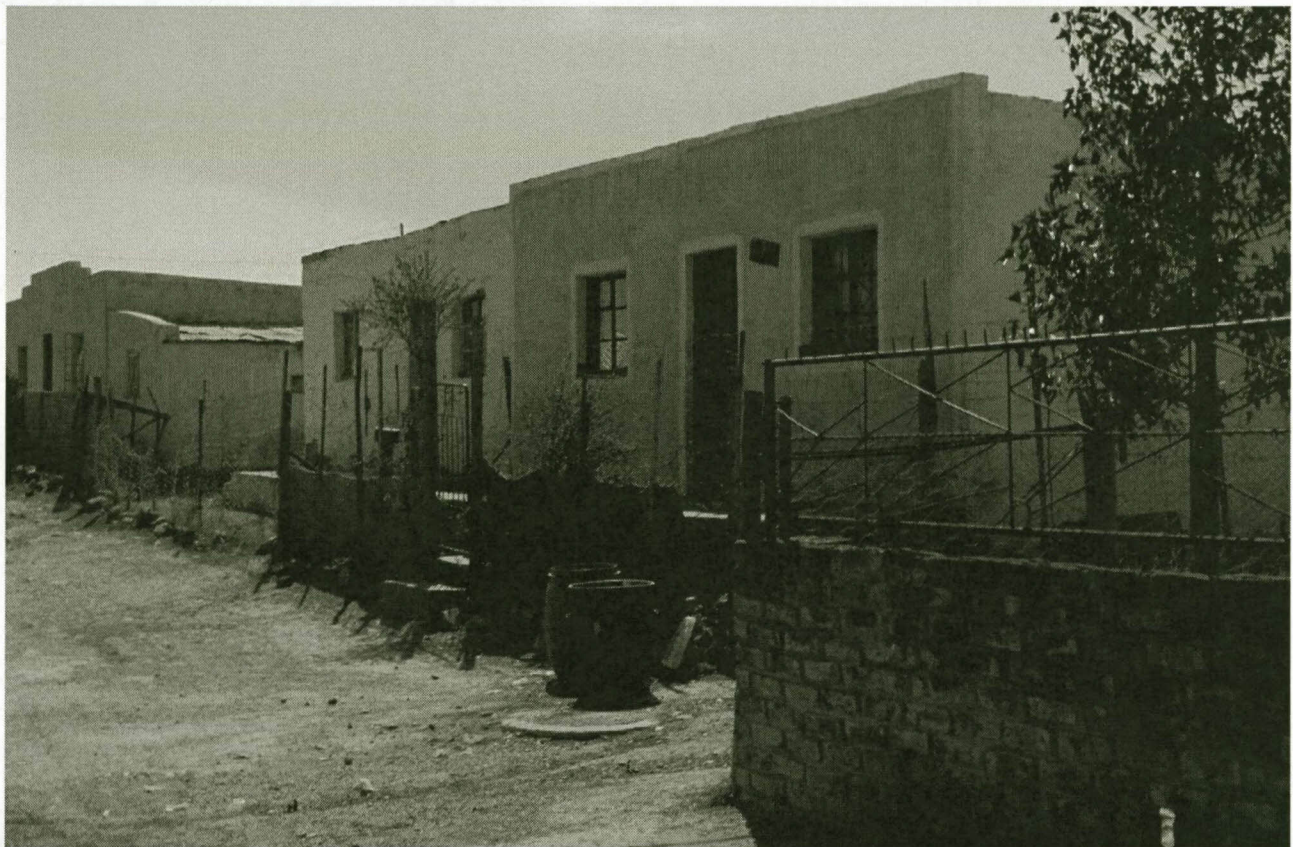
Figure 3.5: Highveld, flat-roofed or brakdak houses found within uMasizakhe
