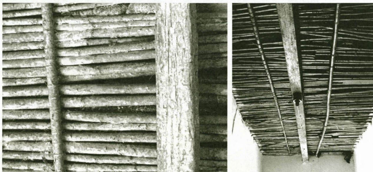
Figure 4.6: Vernacular ceilings of mats of woven reeds placed on rafters
