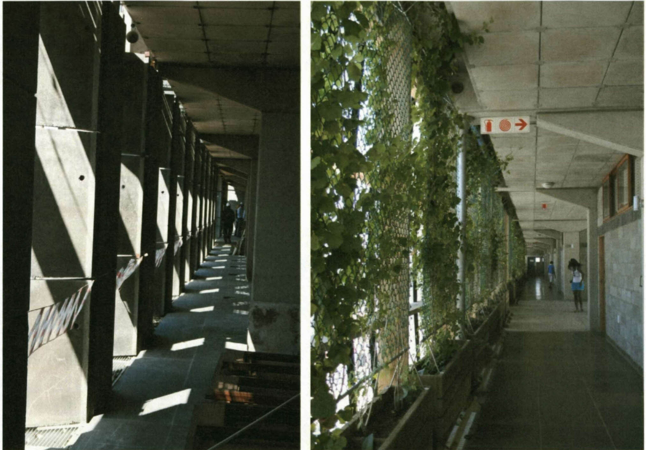
Figure 4.37: Comparative images during construction in 2010 and the completed project in 2012
