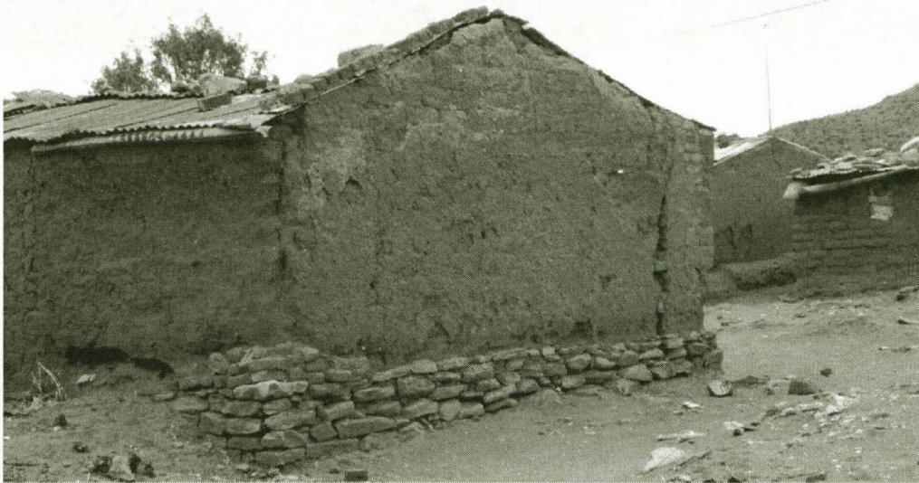
Figure 4.14: A roughly-coursed stone plinth that raises the dwelling, with adobe blocks atop, acting as monolithic structure
