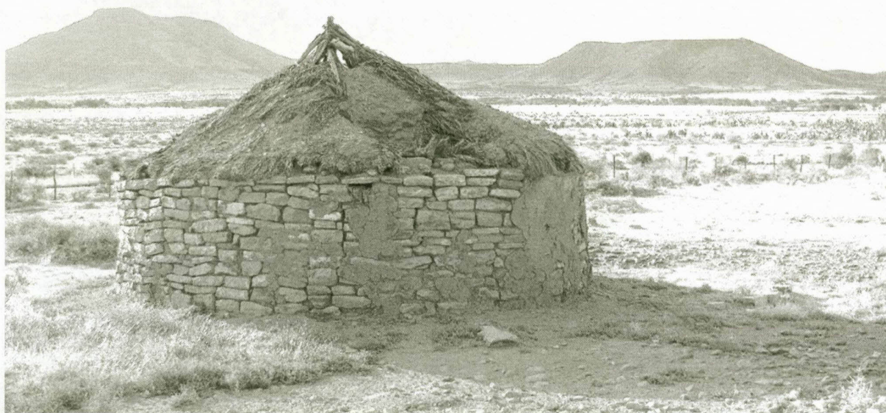
Figure 4.21: Uninhabited and unmaintained R391 rondavel with remaining structural form and roughly-coursed stonework with dagha plaster
