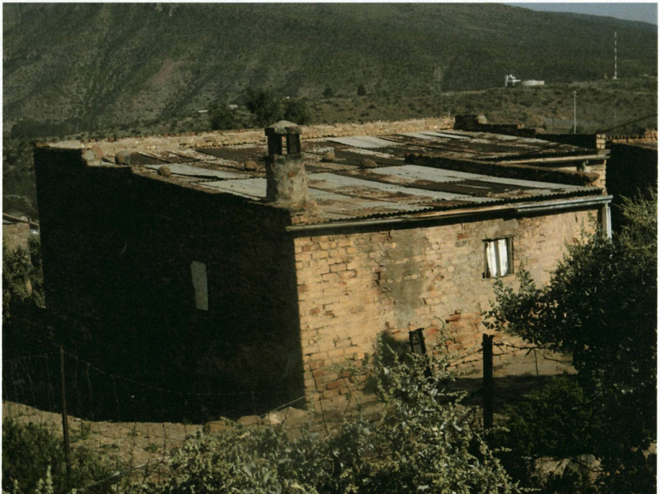
Figure 4.7: The use of corrugated iron on a traditional-vernacular house
