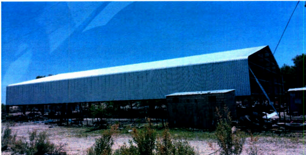
Figure 5.14: Commercial warehouse under construction on a plot of land obtained illegally in the Oshitayi area
