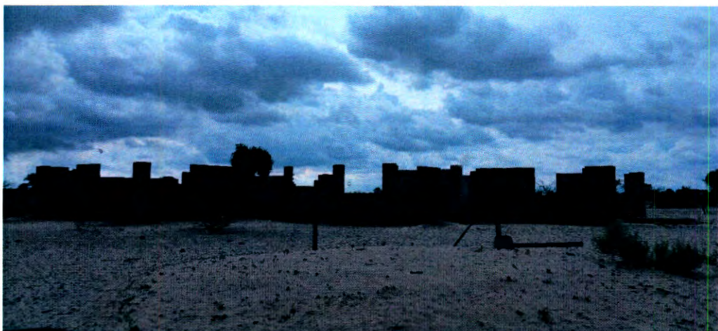
Figure 5.16: A formal brick house under construction on a plot of land obtained illegally in the Oshitayi area
