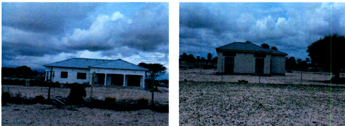
Figure 5.18: High value brick houses under construction on plots obtained illegally in the Oshitayi area
