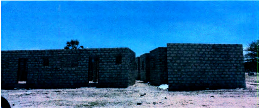
Figure 5.17: Flats under construction on a plot of land obtained illegally in the Oshitayi area
