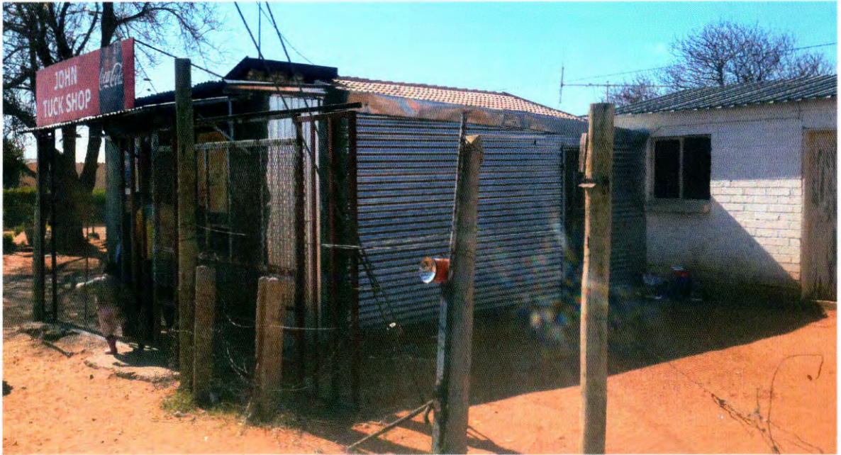
Figure 23: Informal spaza shop in Nobengula Street – structure constructed in front yard of home owner
