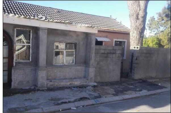
Figure 6.20: Extended house encroaching over the boundary
