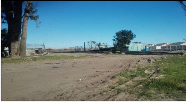
Figure 6.27: Construction site for the further extension of the gap housing Source: Author, 2017
