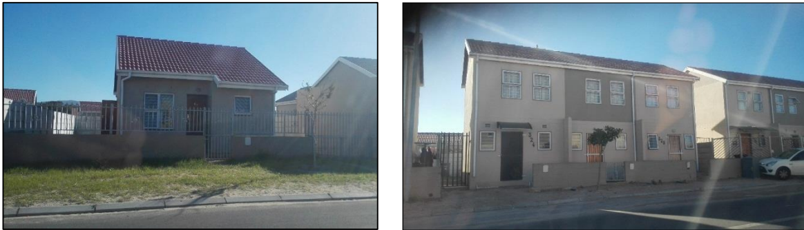
Figure 6.23: Some of the housing typologies throughout the development Source: Author, 2017
