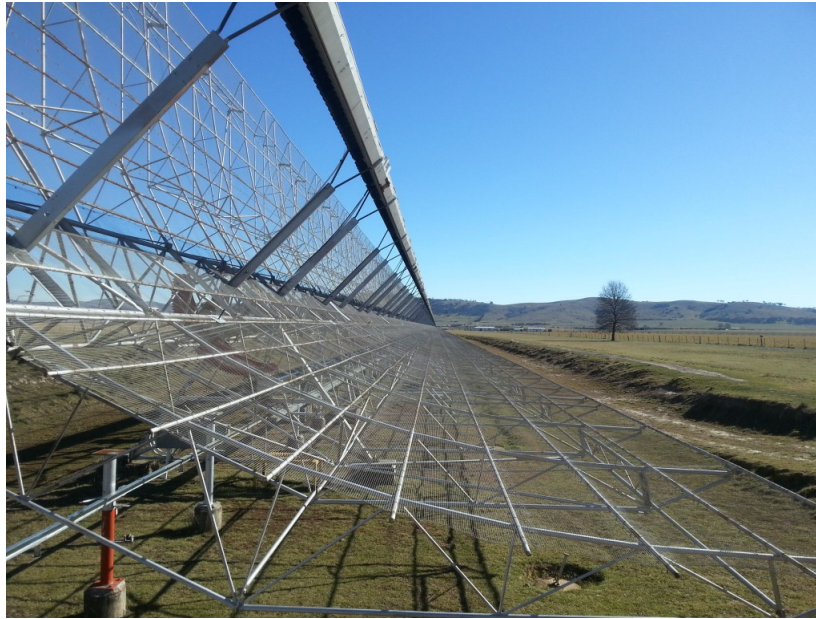
Fig. 5.3: One of the 778m arms of the Molonglo observatory synthesis telescope. Molonglo consist of 352 modules that are individually phased antennae . The modules terminate into 88 receiver boxes within a bandwidth of 100MHz. All the boxes are protected against weather and RFI elements. Pulsars at UTMOST are being timed as part of Molonglo’s TIME project.
