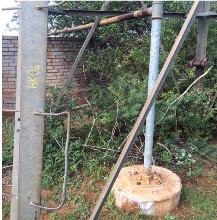
Figure 28: Borehole number on windmill structure
