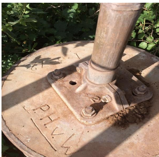
Figure 29a: Hole drilled in base plate
