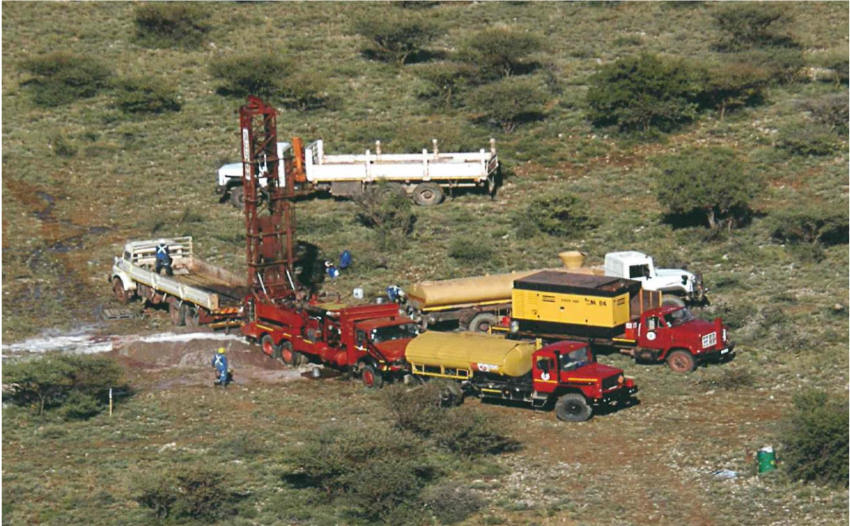
Figure 10: Drilling of boreholes
