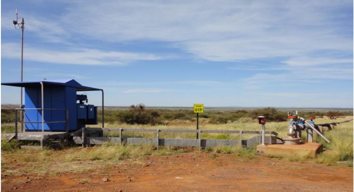
Figure 11: Dewatering borehole connected to dewatering network
