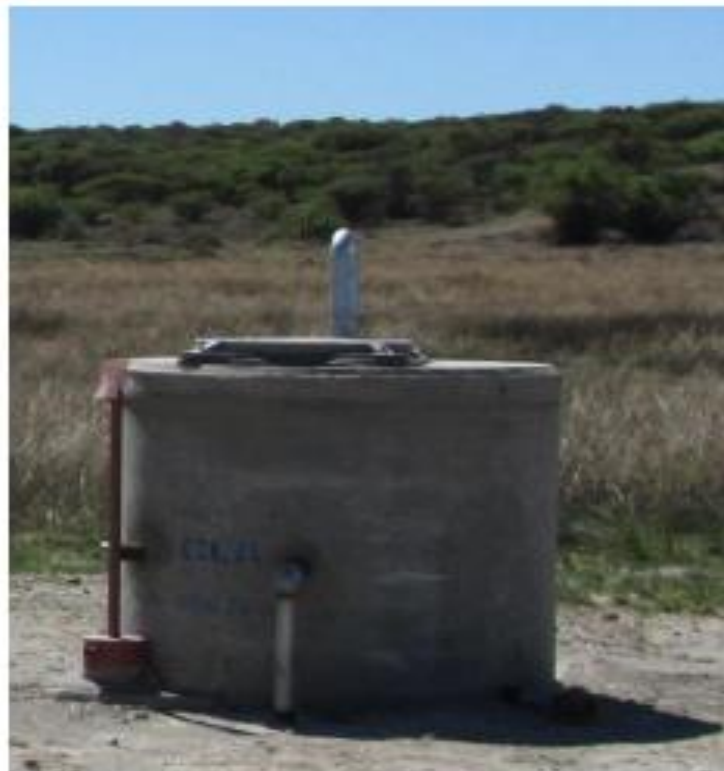
Figure 14: Injection borehole protected by concrete cylinder for artificial recharging of the Groenwaterspruit alluvial aquifer
