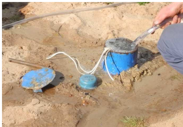
Figure 66: The project team struggling to get the ozonated water into the aquifer due to the bubbling and overflow from the injection well-point
