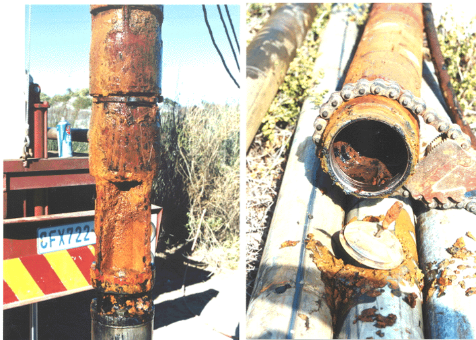
Figure 36: Severe clogging of production borehole G33104 pump intake (left) and MIC by sulphate-reducing bacteria of the non-return valve in production borehole W34001 (right) (More Water cc., 2002)
