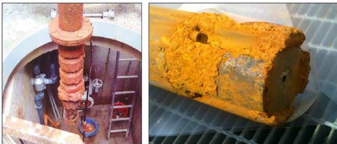
Figure 7: Iron-related clogging of a production borehole (left) and pump (right) in Australia (Deed and Preene, 2013)
