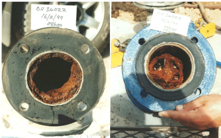
Figure 3: Iron-related clogging experienced at the Atlantis Aquifer of a borehole distribution pipeline between 15-20 mm thick (left) and flow meter (right) (More Water cc., 2002)
