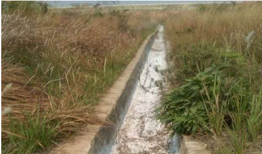
Figure 5-11: Canal from Tailings dam to Return Water Dam
