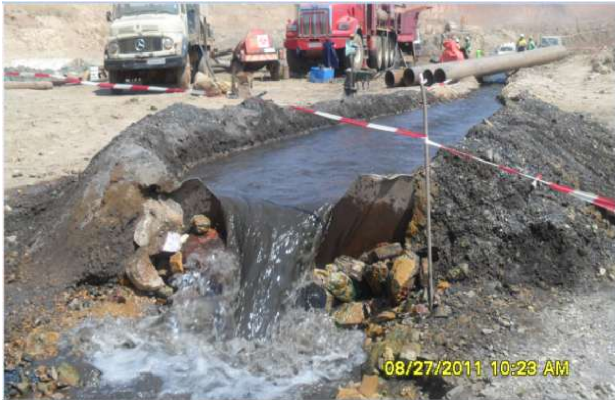
Figure 4-2: Air percussion drilling at dewatering borehole BH1-17 located in Pit 1. The foreground shows passage of groundwater through a V-notch.
