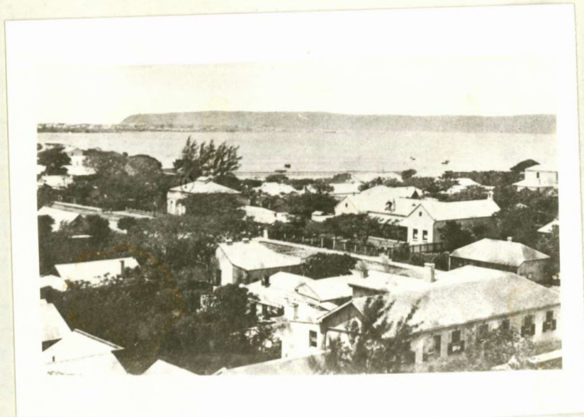
Durban Bay from the former Roman Catholic Cathedral, showing the (1) Masonic Hall and (2) High School in Smith Street.
