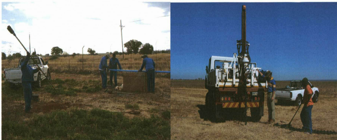
Fig 20: Drilling of the holes
