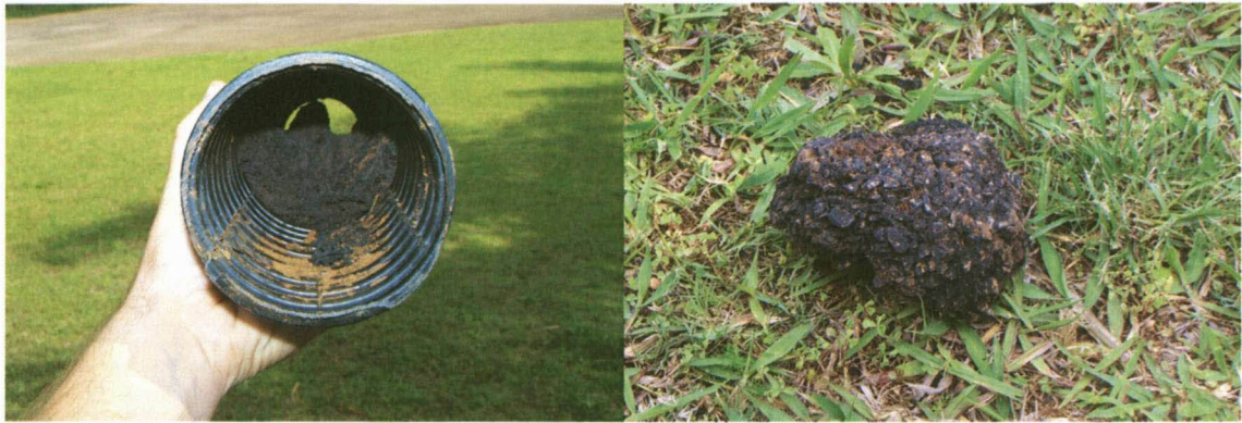
Fig 3: Photo of a blockage recently (May 2009) removed
