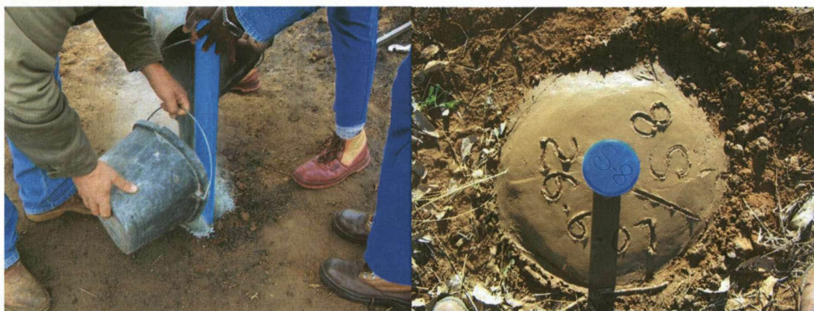
Fig 21: Add filter material and seal the piezometer
