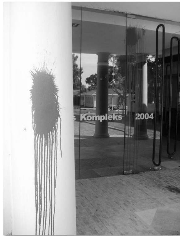
Figure 4.1: Centenary Complex and the Reitz hostel in the reflection
