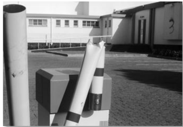
Figure 4.4: Damaged traffic booms
