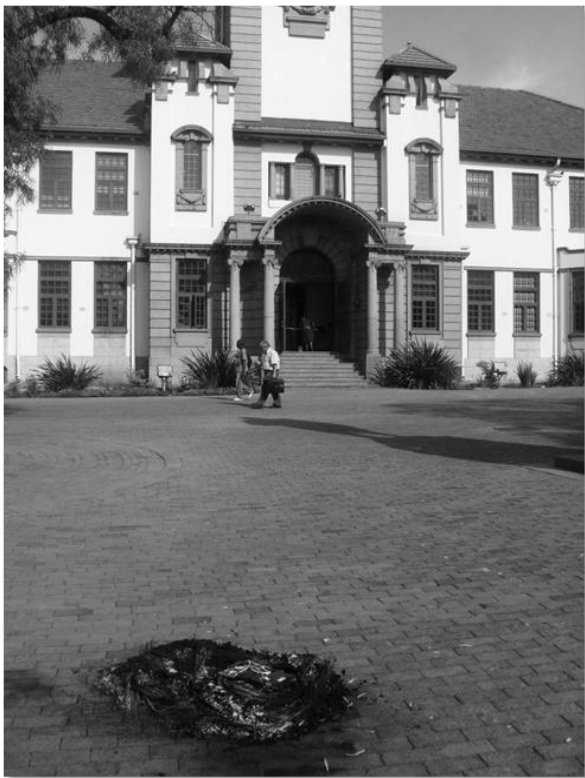
Figure 4.2: UFS Main Building with evidence of destruction in the foreground.
