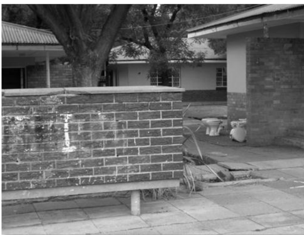
Figure 4.7: The Reitz residence name signage removed.
