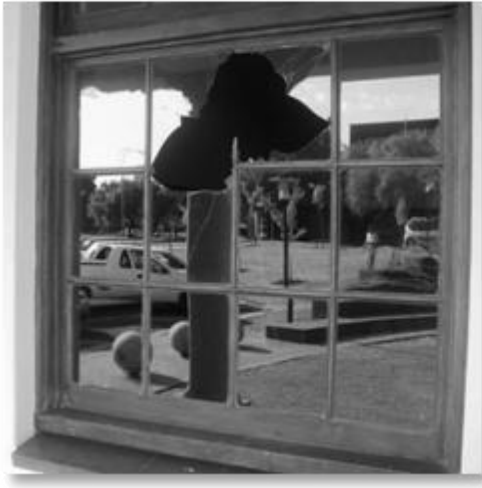
Figure 4.5: Centenary Complex window.
