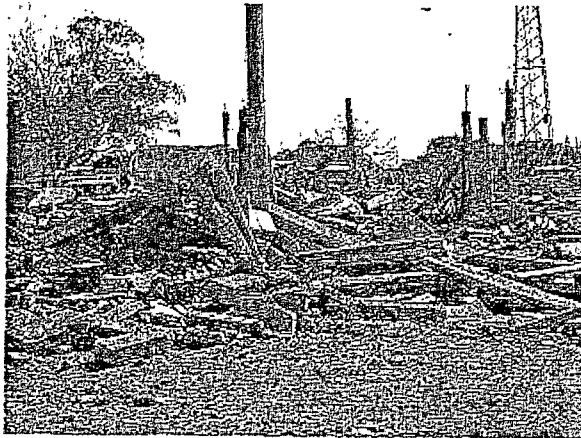
Market stalls demolished in Mbare, Harare.
