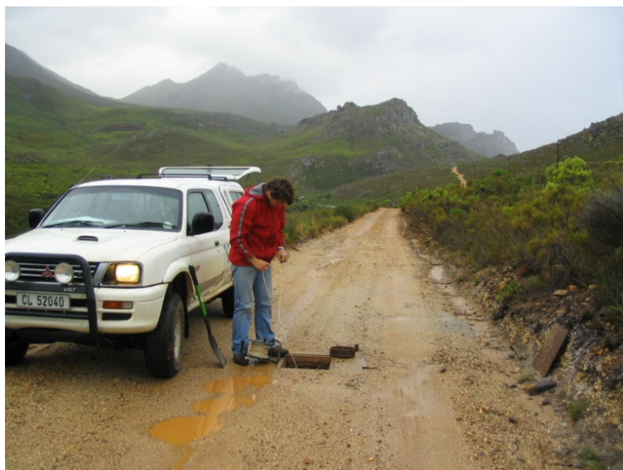
Figure 83. Borehole 1 located in the main access road to the Kogelberg Reserve.
