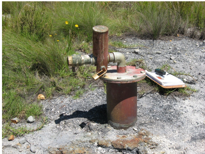
Figure 86. Artesian Borehole 4 located right next to the Oudebosch cottages.
