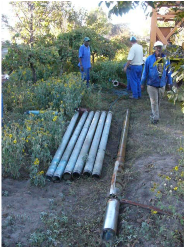
Plate 5. Removal of pump equipment from borehole.
