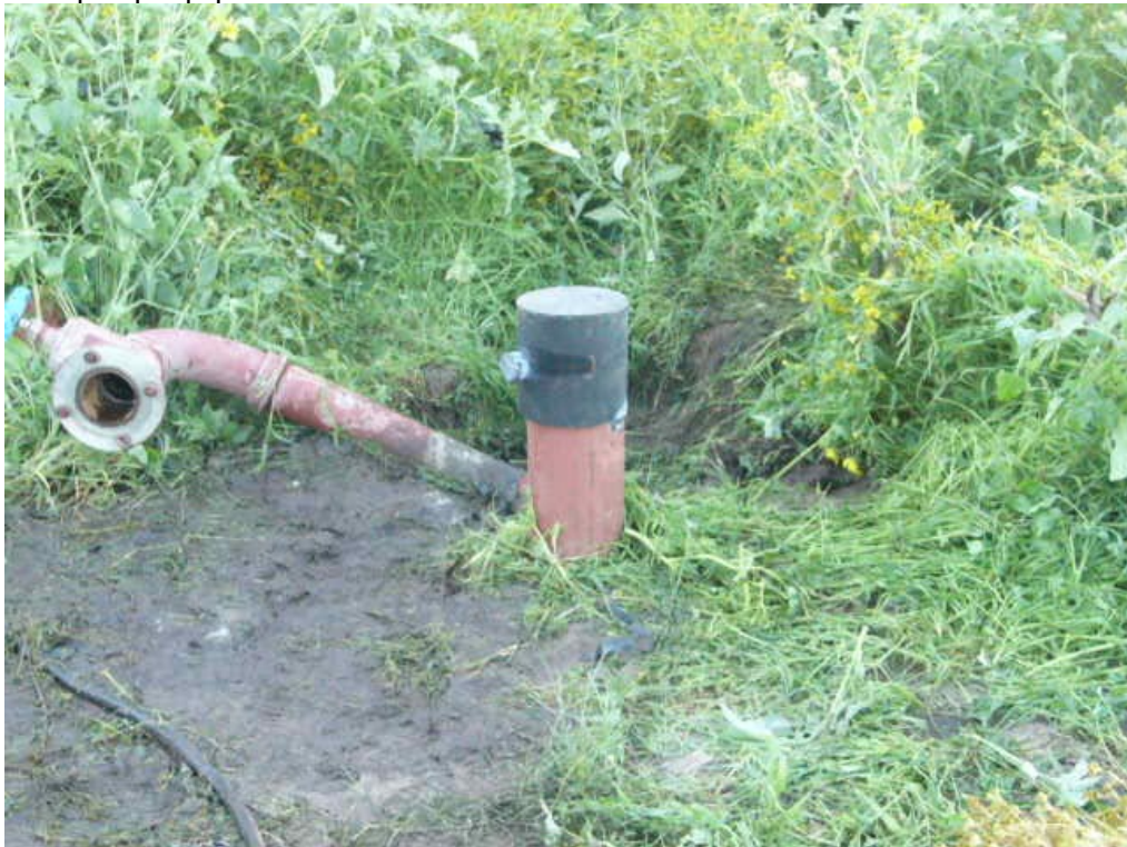
Plate 6. Sealed borehole to enforce compliance.
