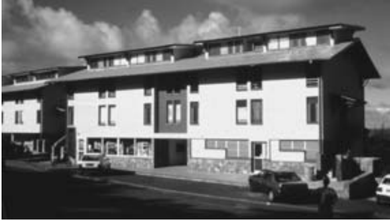
Photo 2: Contemporary three storey block of flats of Compressed Earth Blocks on the Island of Mayotte Source: CRA Terre-EAG library
