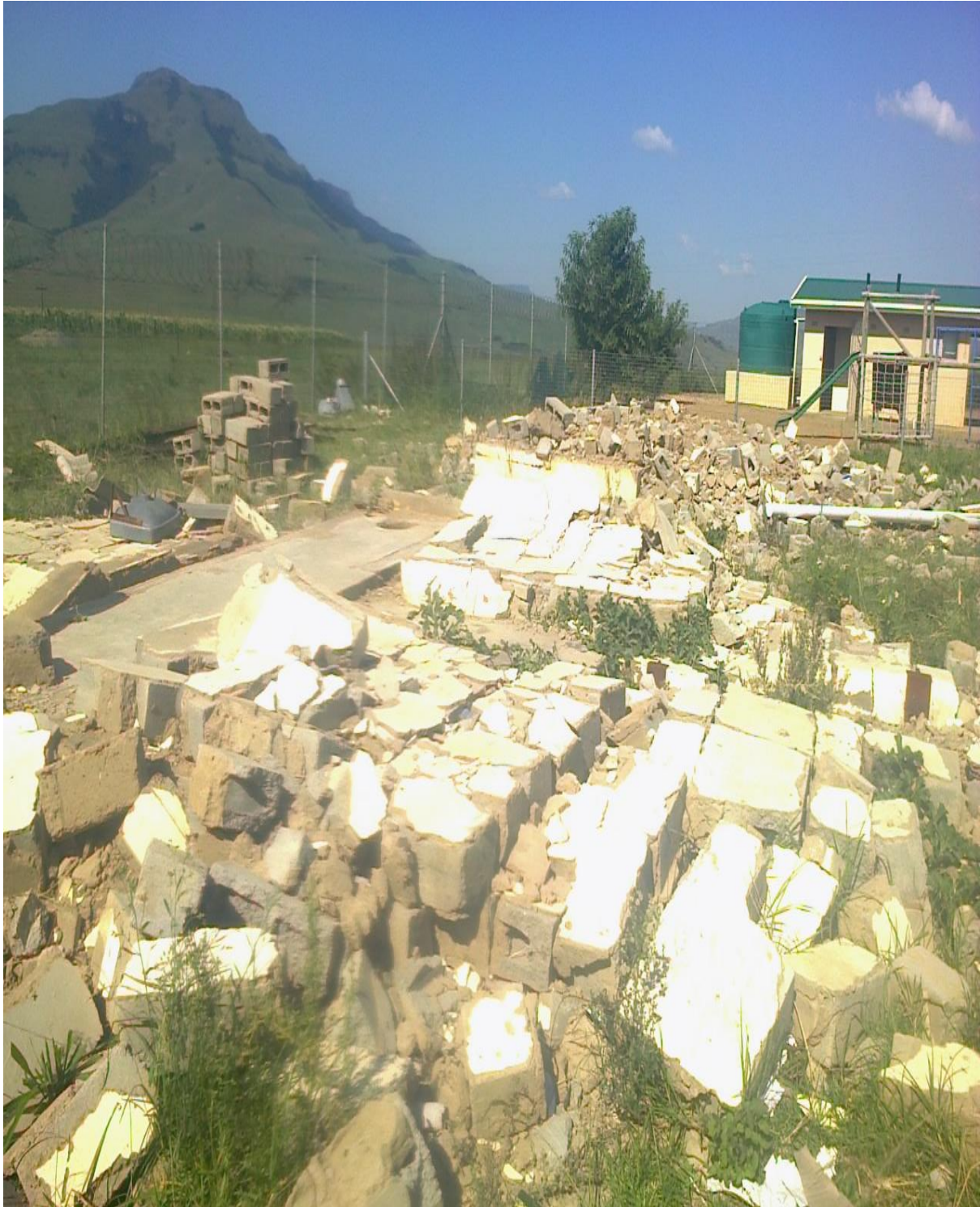
Picture 2. Dangerous rubbles from a collapsed toilet block at Ndlamlenze combined school. Note that the pits were open at the time of the research, posing a danger to learners falling into them while playing.
