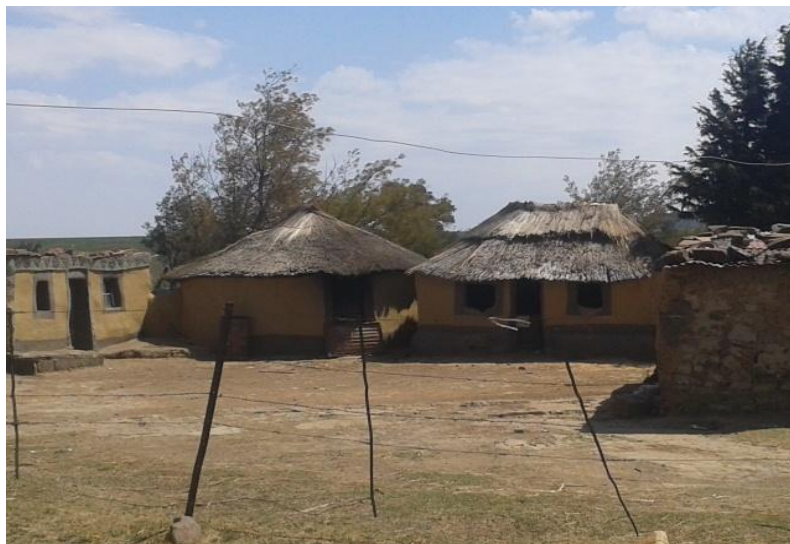
Illustration 5.3 Repaired thatch roof of a beneficiary's dwelling
