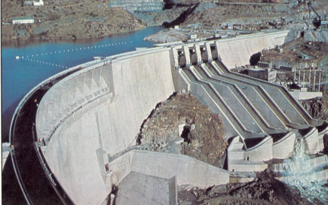
Fig. 1.2 Gariep Dam under construction in 1972
