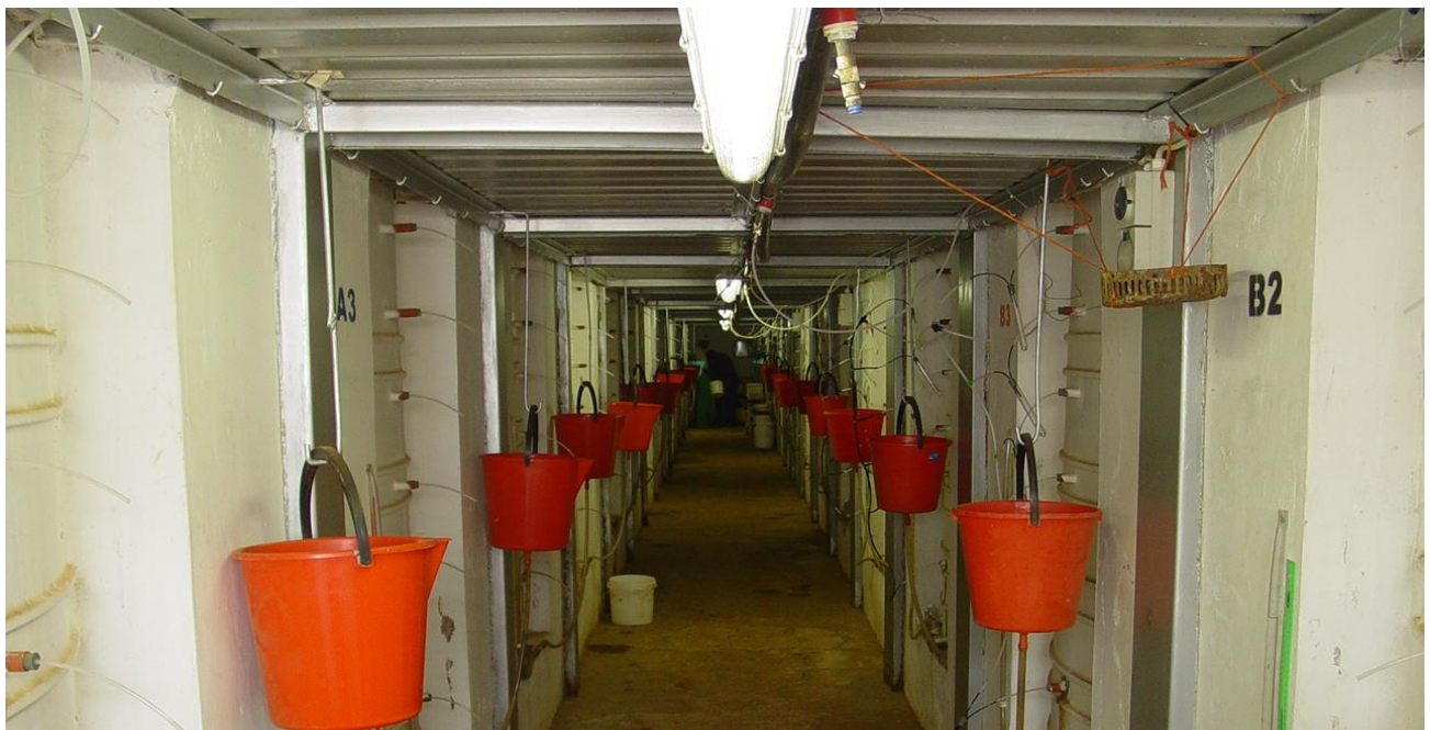
Figure 3.2 Underground chamber with manometers connected to the bottom of each lysimeter.
