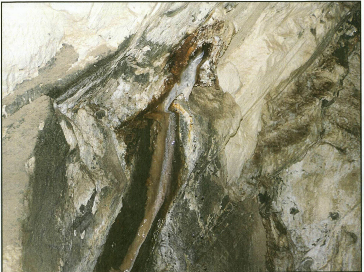
Figure 42: Fault bearing water at Harmony Evander No. 8 shaft 11 level (1340 m below surface).
