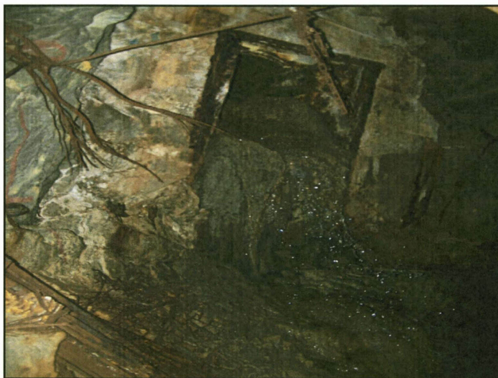
Figure 16: Groundwater flowing into the gold mine via exploration borehole in a gold mine shafts.
