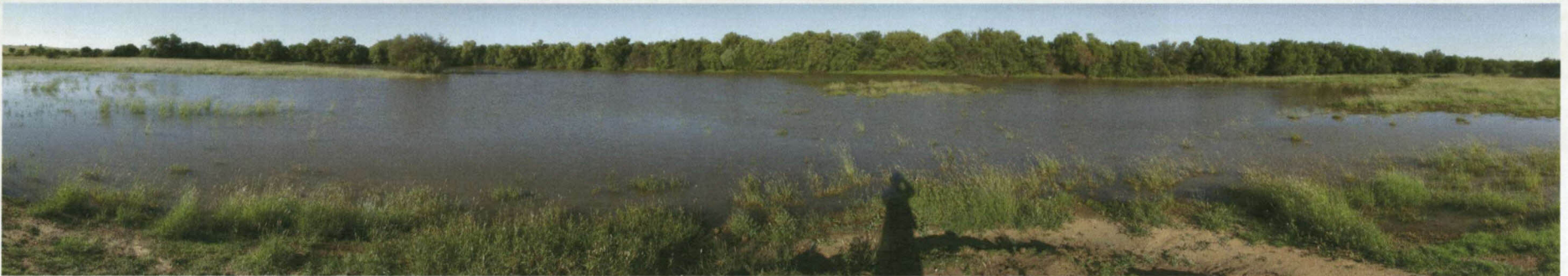
Figure 2.9: Contrasting conditions at the farm dam in the drainage line at Glen.
