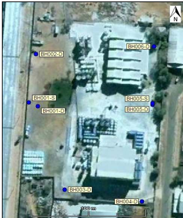
Figure 15: Aerial map of the SNP site indicating the locations of the boreholes.
