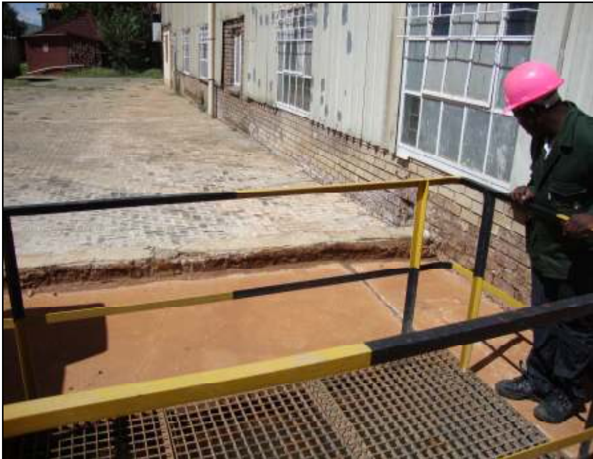
Figure 39: Photo indicating the chemical damage to the pavement and building on the northern side on the SNP plant.
