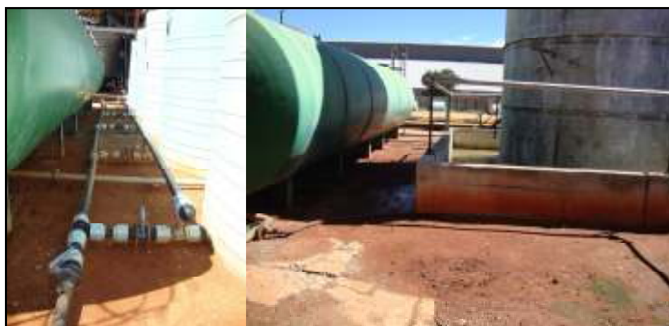
Figure 42: Photos of storage tank area in the centre of the site.
