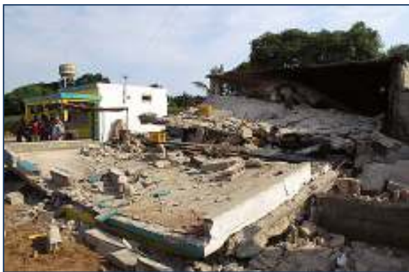
Figure 1.7 Demolished buildings in Maputo
