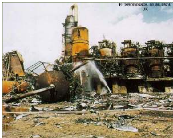
Figure 1.11 Destruction at the Nypro plant in Flixborough
