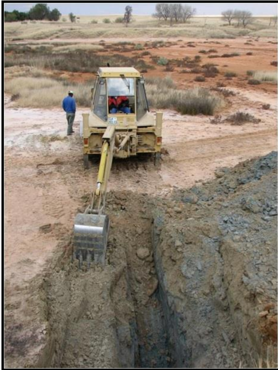
Figure 11.6: Trench 3 being excavated.
