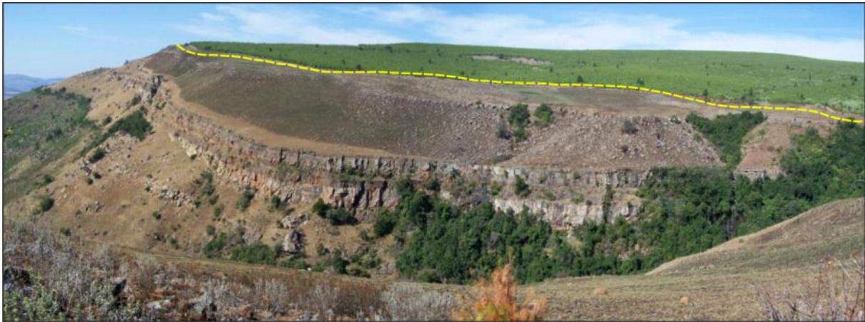
Figure 5.12: The landscape picture above shows the central body of the HMS-1 (view in SSE direction). The yellow dashed line marks the contact with the Timeball Hill Shale. Notice the different Klapperkop Quartzite layers below the Timeball Hill Shale.
