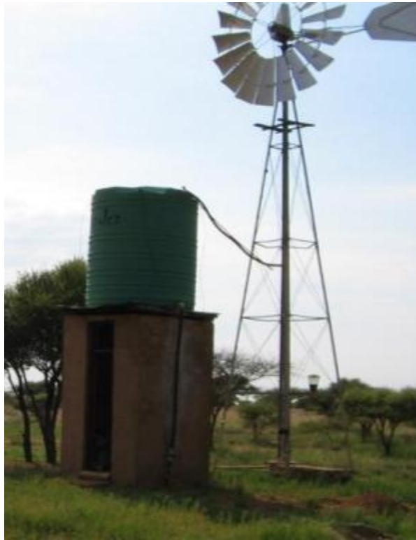
Figure 13: Wind pump used primarily for live stock watering
