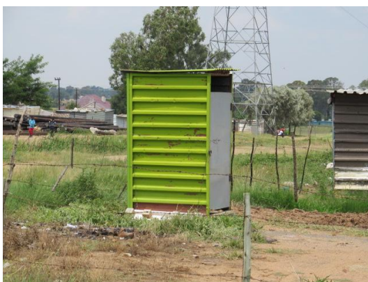
Picture 6.11: Toilet structure built around a pit
