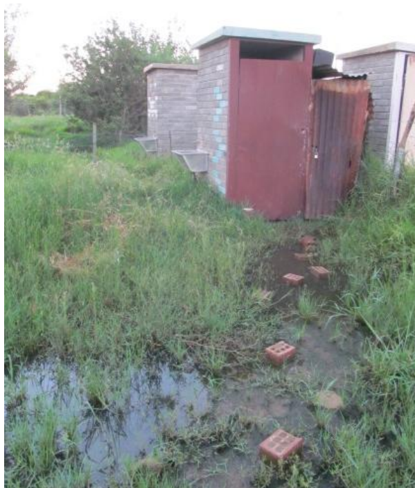
Picture 6.5: Sewerage leaking from a toilet
