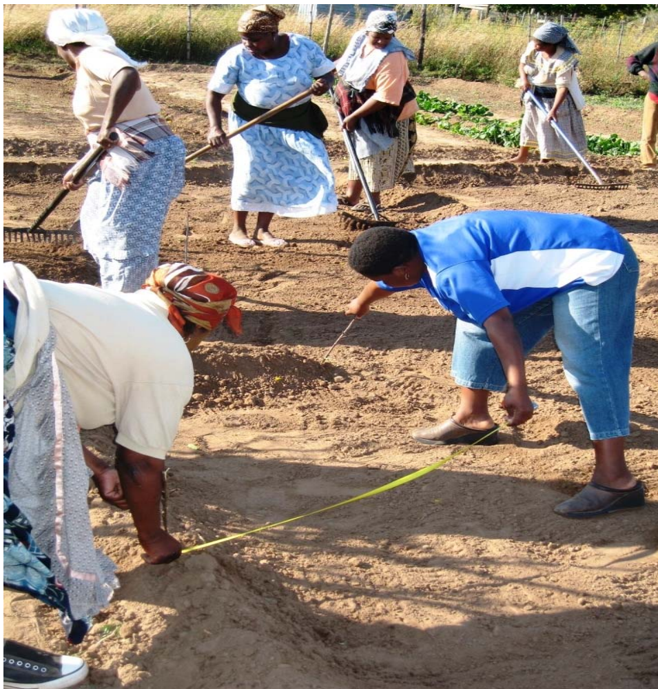
Photo 4.2 Women working together to construct the IRWH crop bed (Source: ARC-ISWC)
