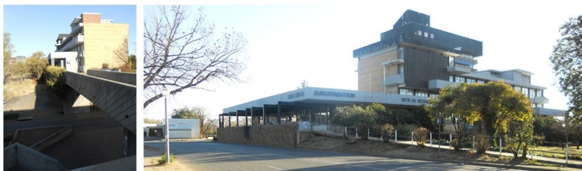
Figure 43. Sasolburg civic centre, Sasolburg. A: The ramp connecting the centre with the public library. B: Access to the centre provided by a ramp which is isolated from the street.
