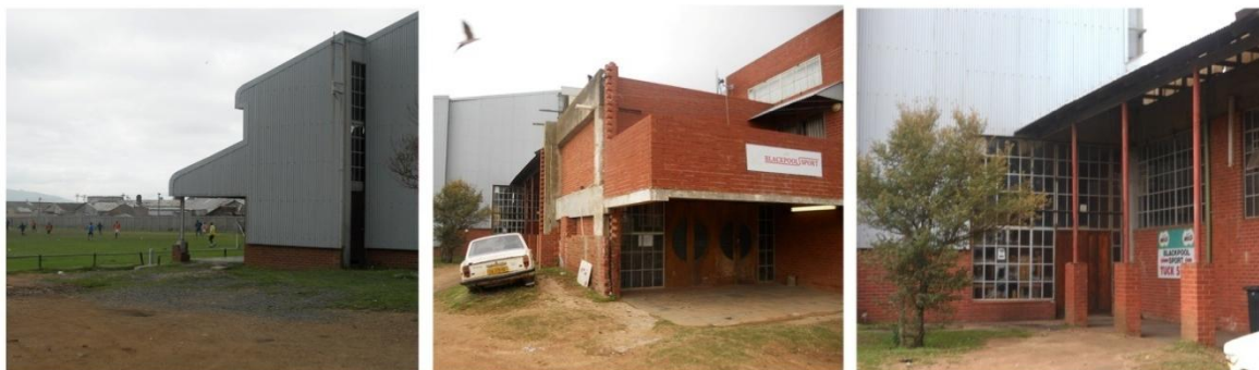
Figure 46. Salt River community centre, Cape Town. A: Adjacent to the sports field is the covered veranda for spectators. B: The entrance with a rentable unit for the care taker in a run-down state. C: The entrance to the central multi-purpose gathering space.
