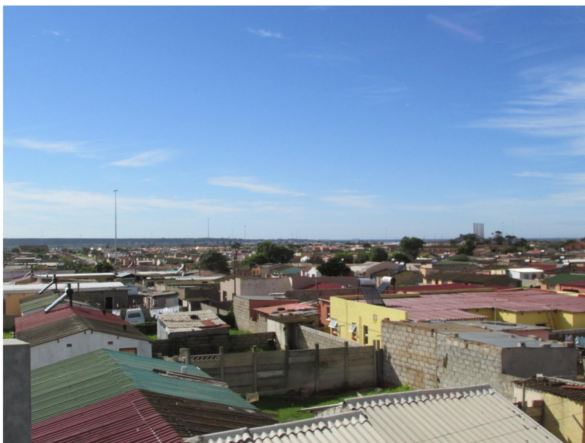
Figure 30. Houses adjacent to Qeqe Street as seen from Ubuntu's rooftop. Note the additions to the original duet units.
