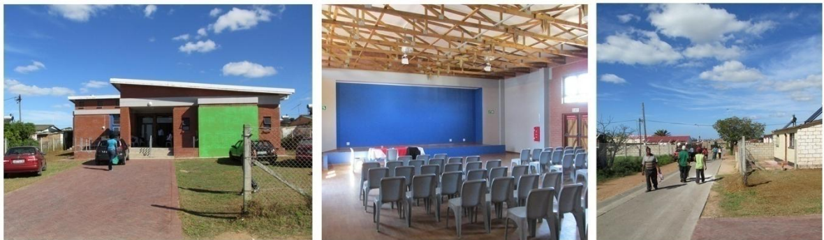
Figure 59. Zwide community hall, Port Elizabeth. A: The entrance of the Zwide hall as seen from the street. B: The small gathering space provided. C: Access to the centre is provided from a secondary street.
