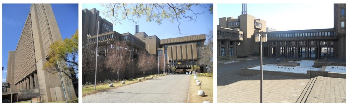
Figure 42. Johannesburg civic centre, Johannesburg. A: The administrative section of the civic centre. B: The civic centre positioned in a park environment. C: Public space is provided although the scale remains inhuman.
