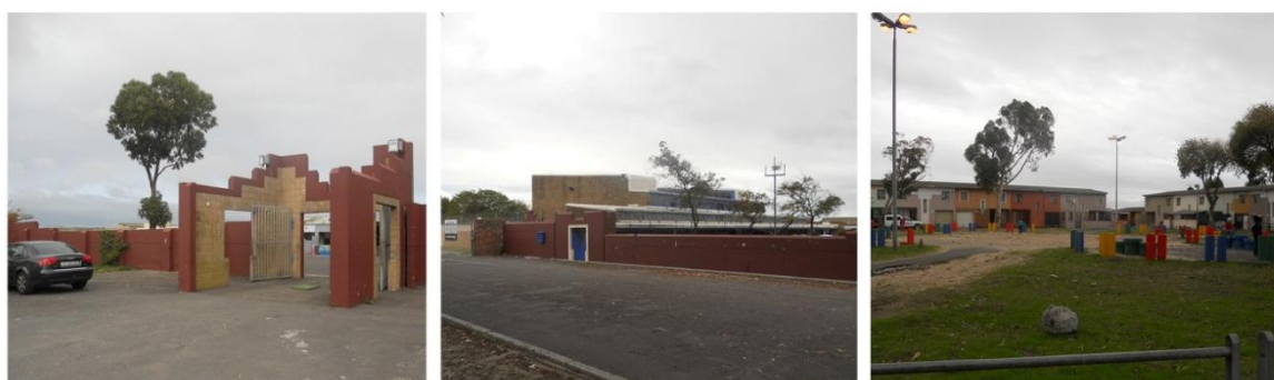
Figure 45. Belhar community hall, Belhar. A: The entrance to the centre altered for vehicle access. B: The boundary wall surrounding the community hall restricting visual access. C: The more open public play area opposite the Belhar hall.
