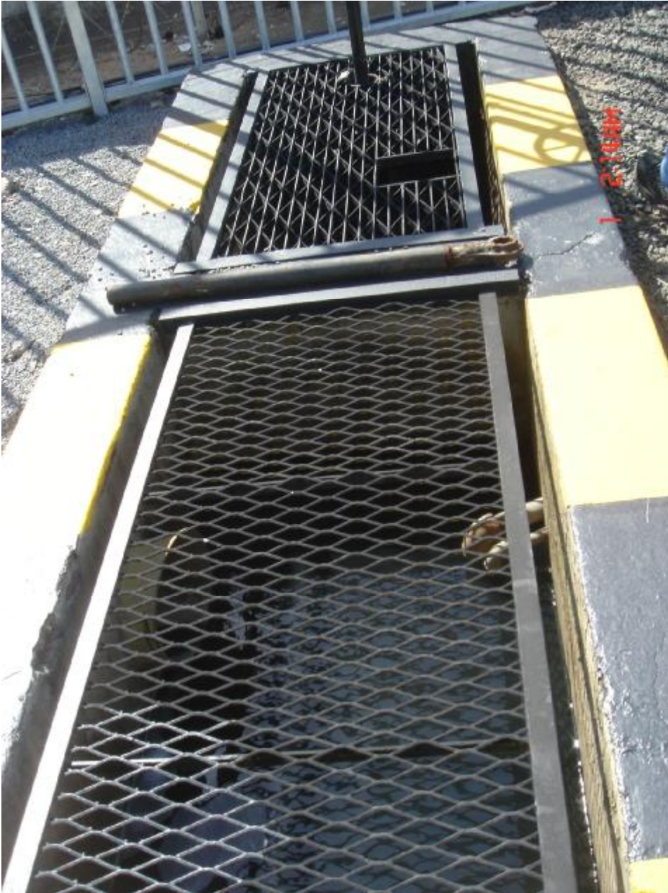
Figure 76: Oil separator and run-off collection pit.
