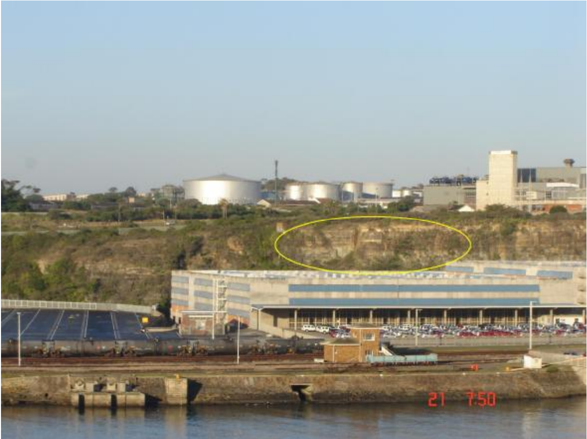
Figure 40: Geology below the project area. Tank farm can be seen in the background.
