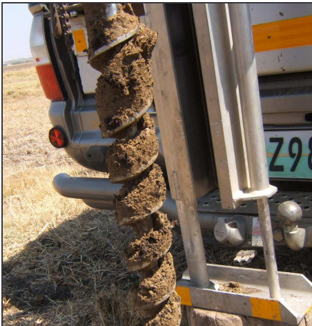
Figure 16: Auger solid stem drilling at the landfill site.
