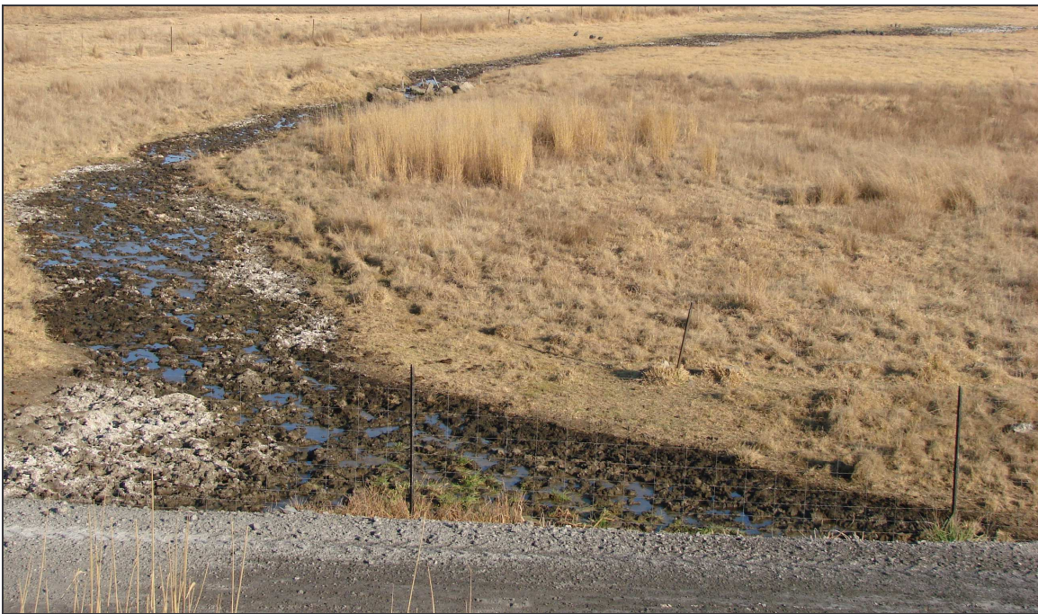
Figure 35: Seepage flow (contaminated canal) from leachate springs west of the Charlie I landfill site.
