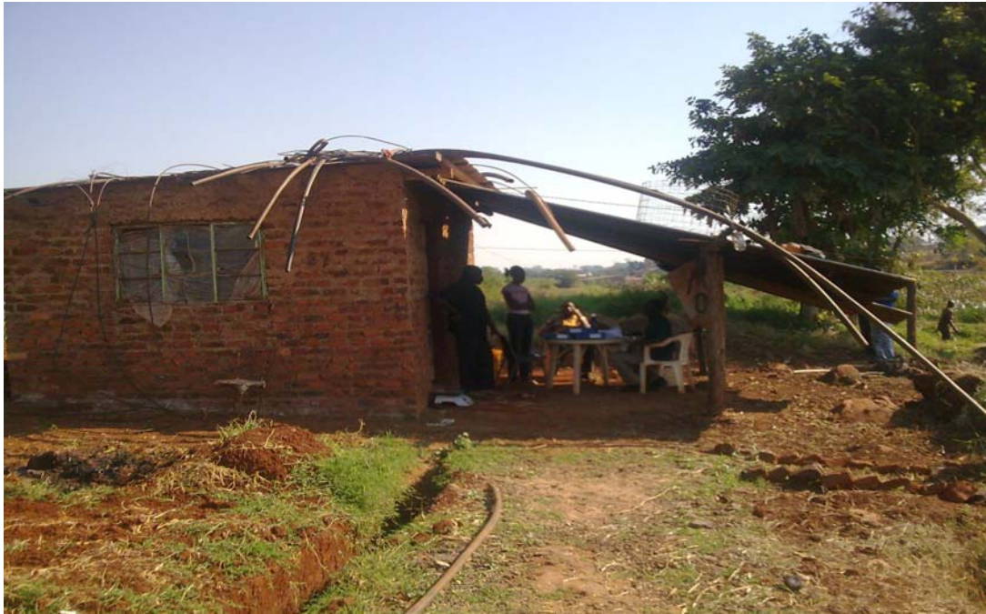
Picture 1 Office facility for small-scale enterprise in Limpopo
