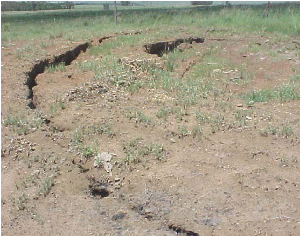
Figure F: Surface subsidence and prior rehabilitation above a stooped area
