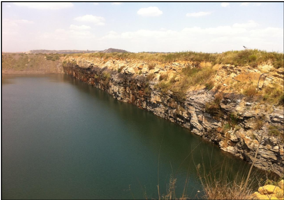
Figure 1: Klipspruit mine pit, where water is seeping into the pit.
