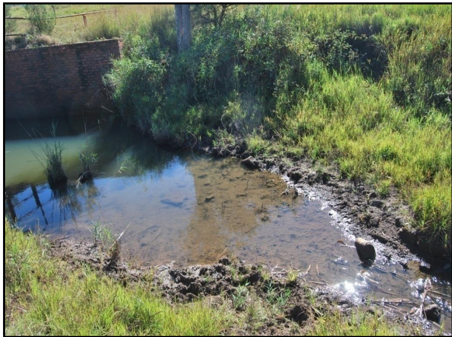
Golf dam downstream.
