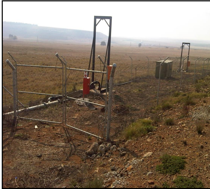
Figure 52: Photograph of the extraction wells pumping water from Usutu South to Mooiplaats Colliery.
