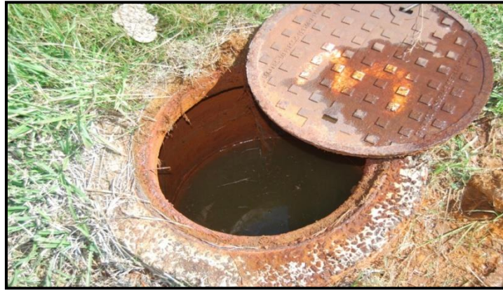
Figure 103: Photograph of KMH3.
