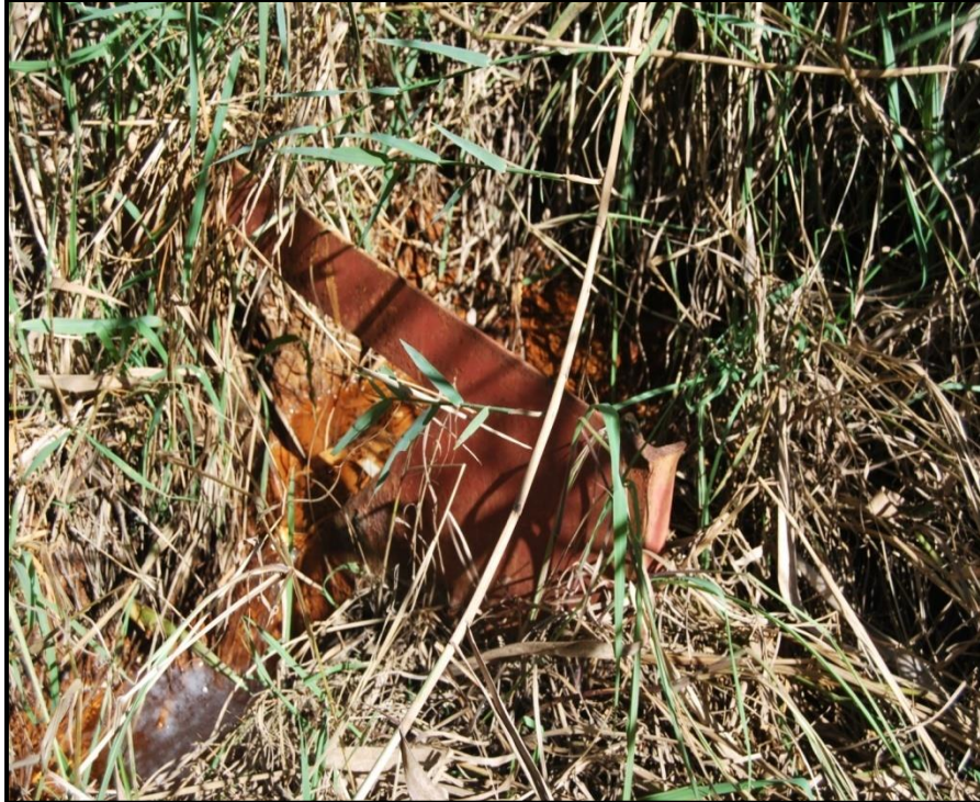
Village stream V-notch
