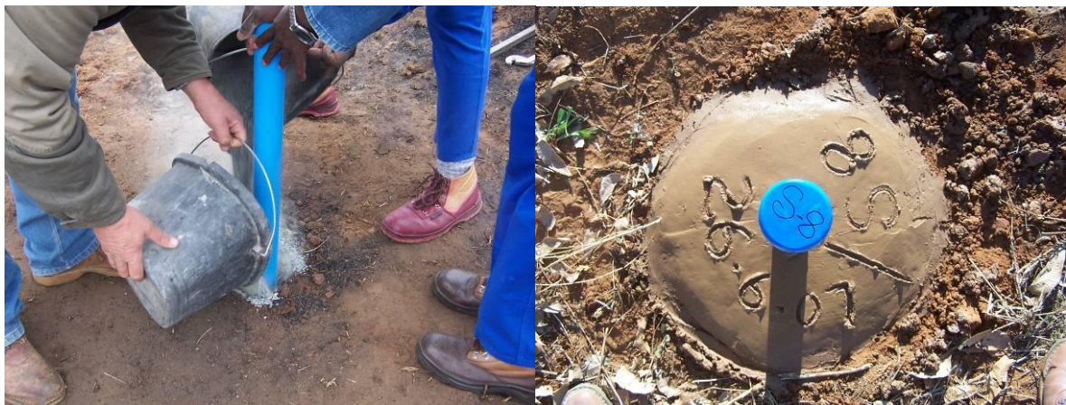
Fig 21: Add filter material and seal the piezometer
