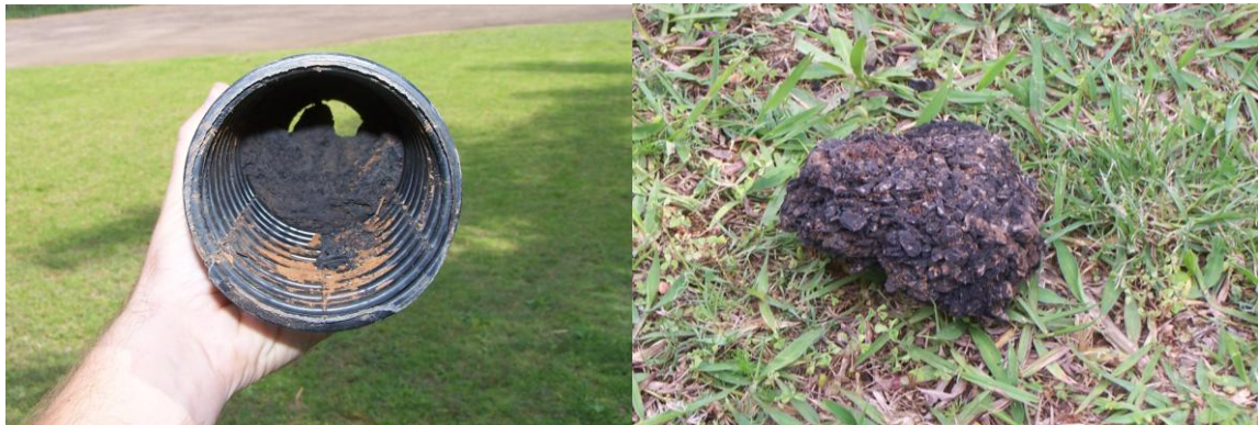
Fig 3: Photo of a blockage recently (May 2009) removed
