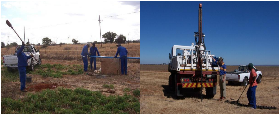
Fig 20: Drilling of the holes
