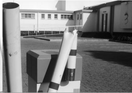
Figure 4.4: Damaged traffic control booms.
