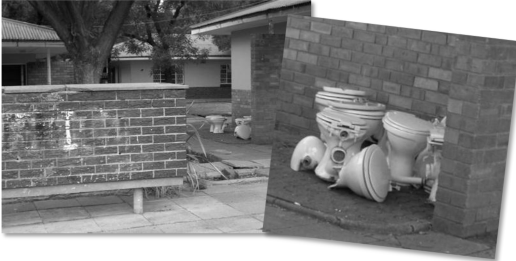
Figures 4.7: Renovations at the Reitz hostel.
