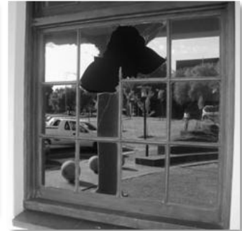
Figure 4.5: Centenary Complex window.
