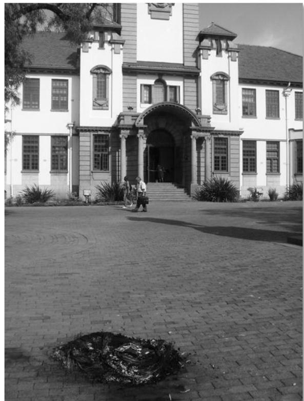
Figure 4.2: UFS Main Building with evidence of destruction in foreground.
