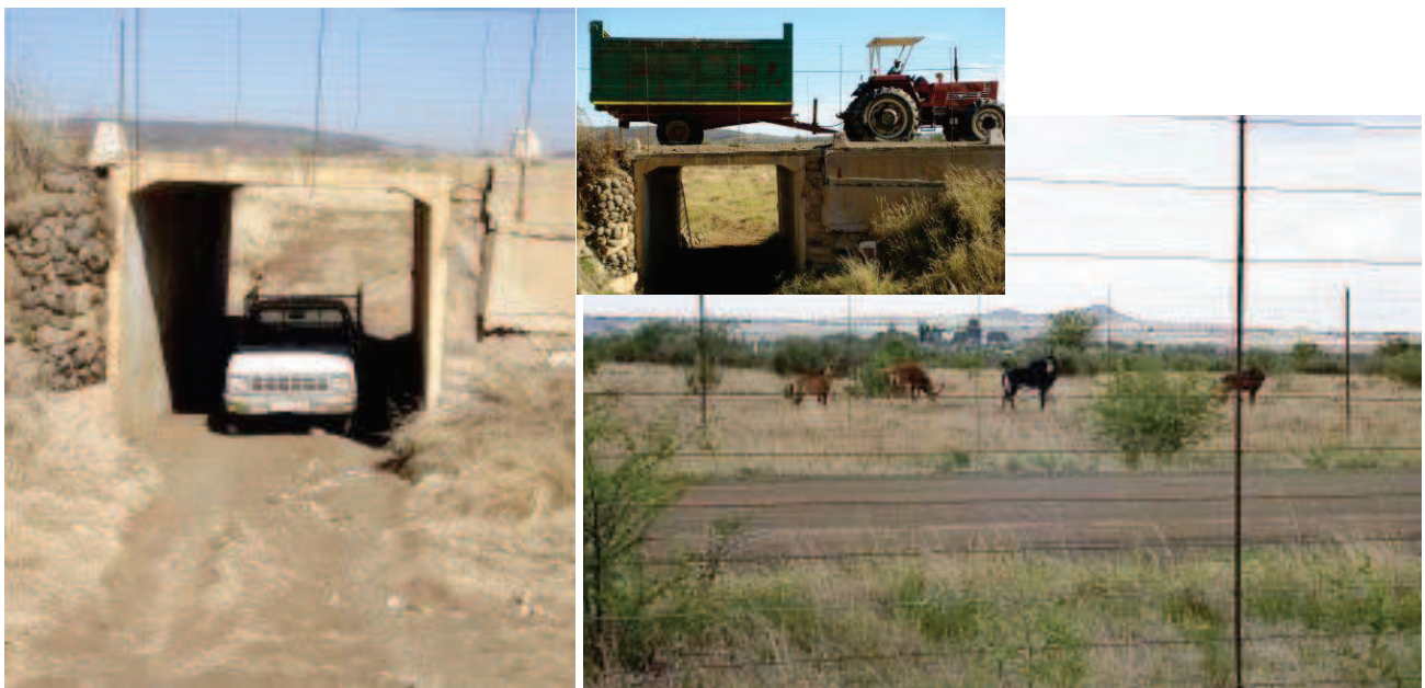
Figure 3.2 The gravel road to Soutpan divides the reserve into two parts with a connecting tunnel underneath the road that allows limited passage of game between sides. The vehicle indicates the size of the tunnel.
