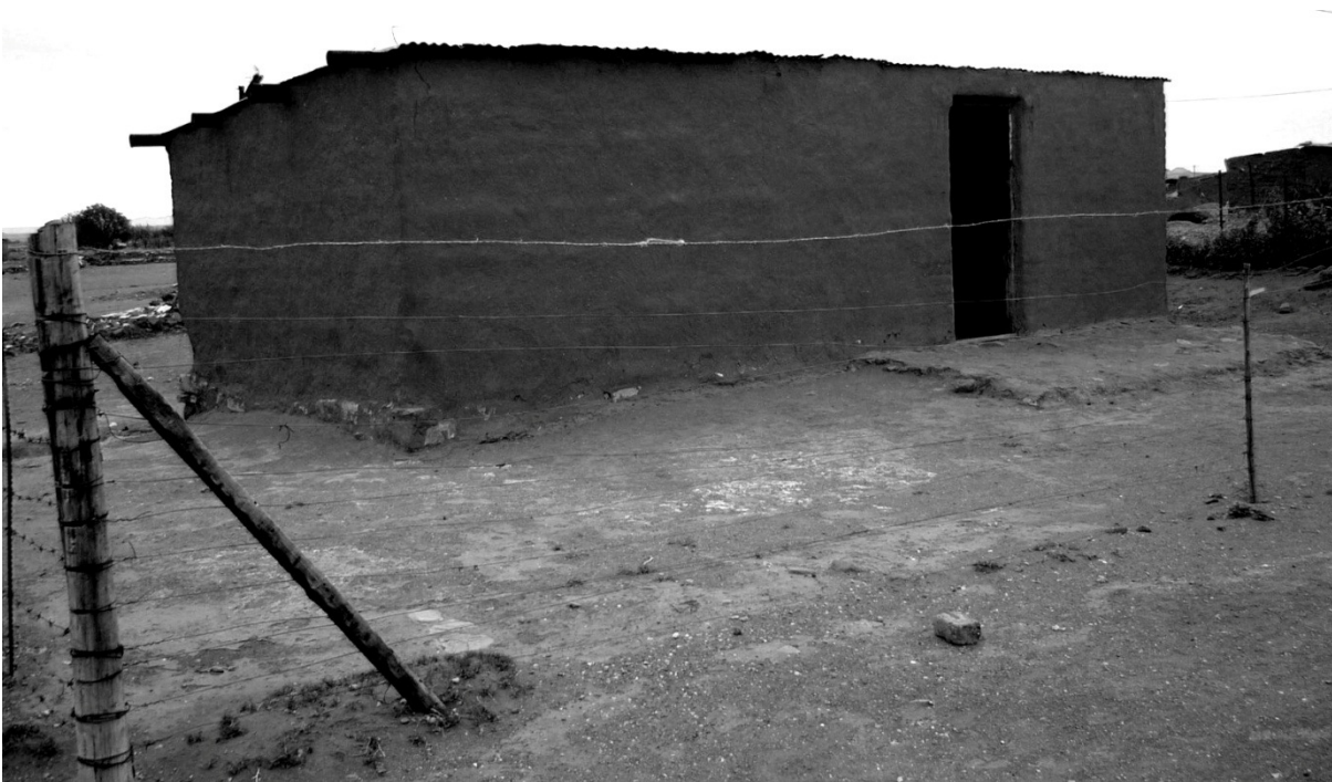
Figure 4.16: A well maintained adobe dwelling with plinth of available rubble and slightly raised threshold for preventing storm water from entering dwelling
