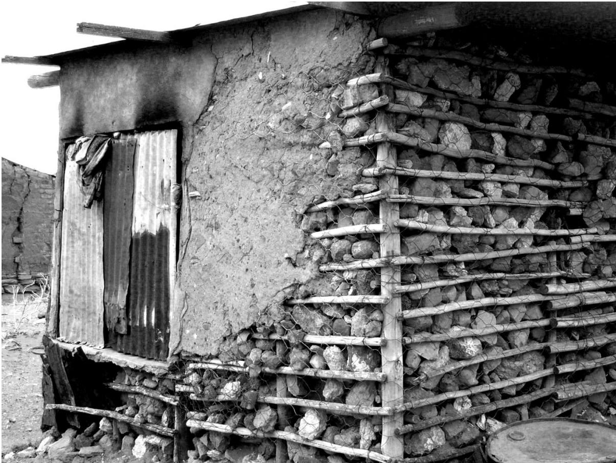
Figure 4.12: An open-order timber frame structure with double-sided laths and wire mesh used to contain the rubble infill in place
