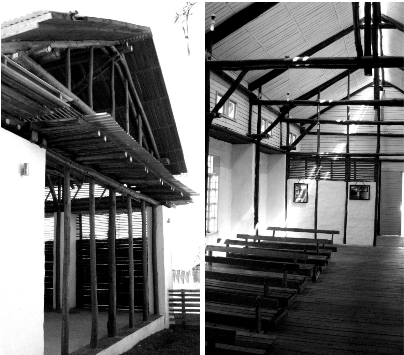
Figure 4.28: GFSC's Chief's Hall with wattle and daub walls and site-sourced timber together with the use of natural light and contemporary innovative design
