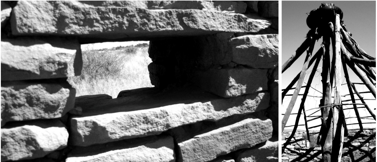
Figure 4.25: Notice the horizontal stone acting as a lintel for the small window opening (left), and tyre that holds together the radiating rafters (right)
