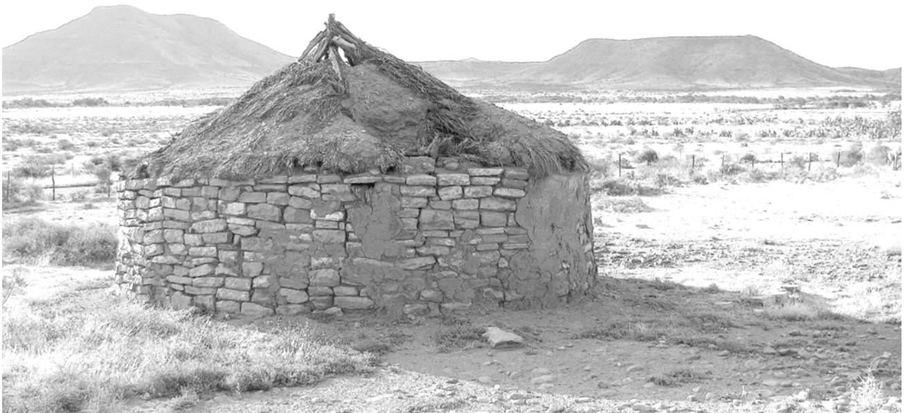
Figure 4.21: Uninhabited and unmaintained R391 rondavel with remaining structural form and roughly-coursed stonework with dagha plaster
