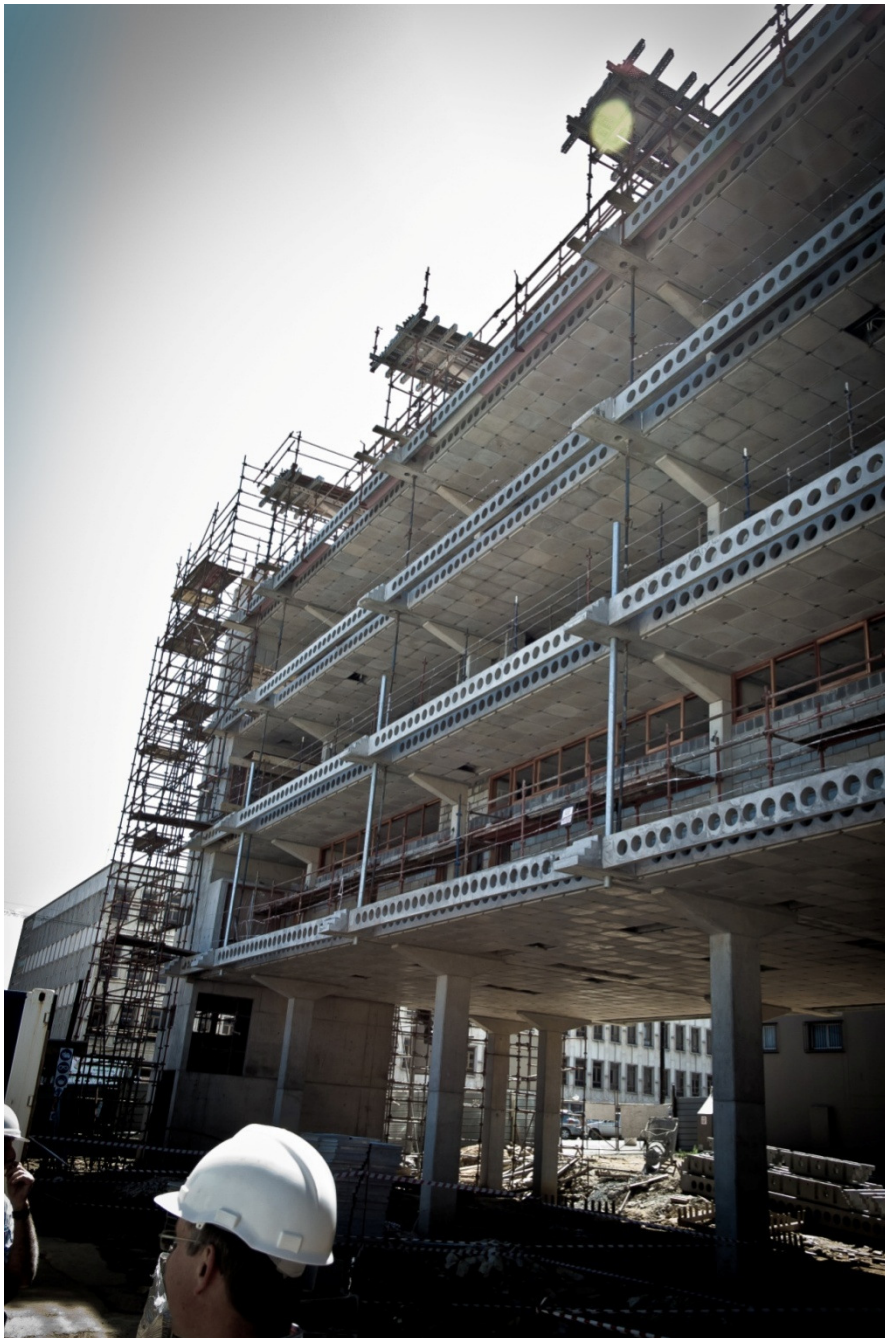
Figure 4.34: Image of the construction process in 2010 with precast beams and ceiling visible
