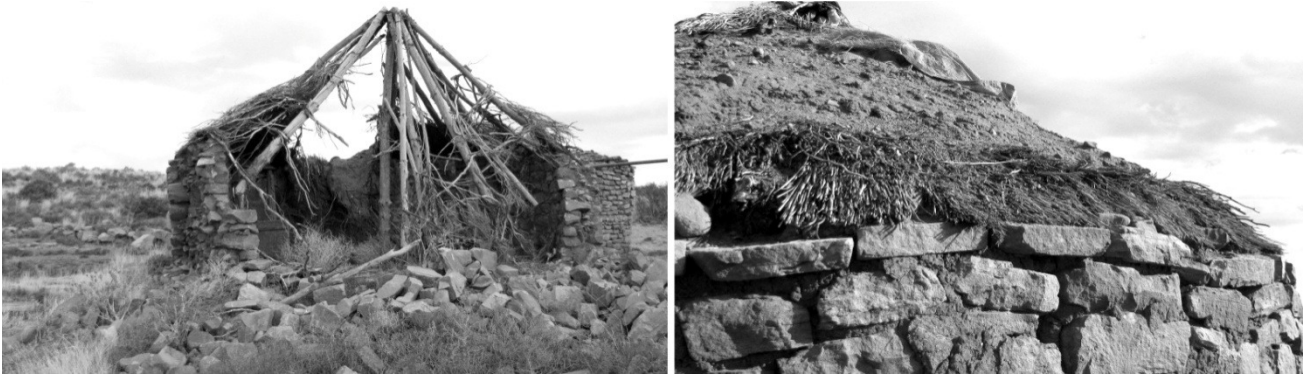
Figure 4.22: Thick, coarsely laid stone walls and centre post providing structural integrity to the rondavel (left), and earth and on top of hessian bags on roof limiting earth from seeping into rondavel
