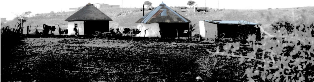
Figure 3.10: Transkei, 2009, the evolution of the dwelling forms from circular to rectangular as a result of the introduction of corrugated iron
