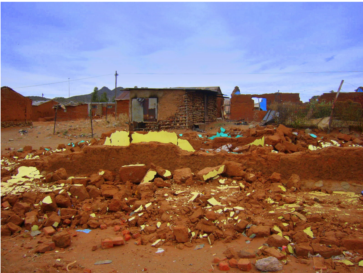
Figure 4.11: A demolished vernacular home in Luxolweni, 2007
