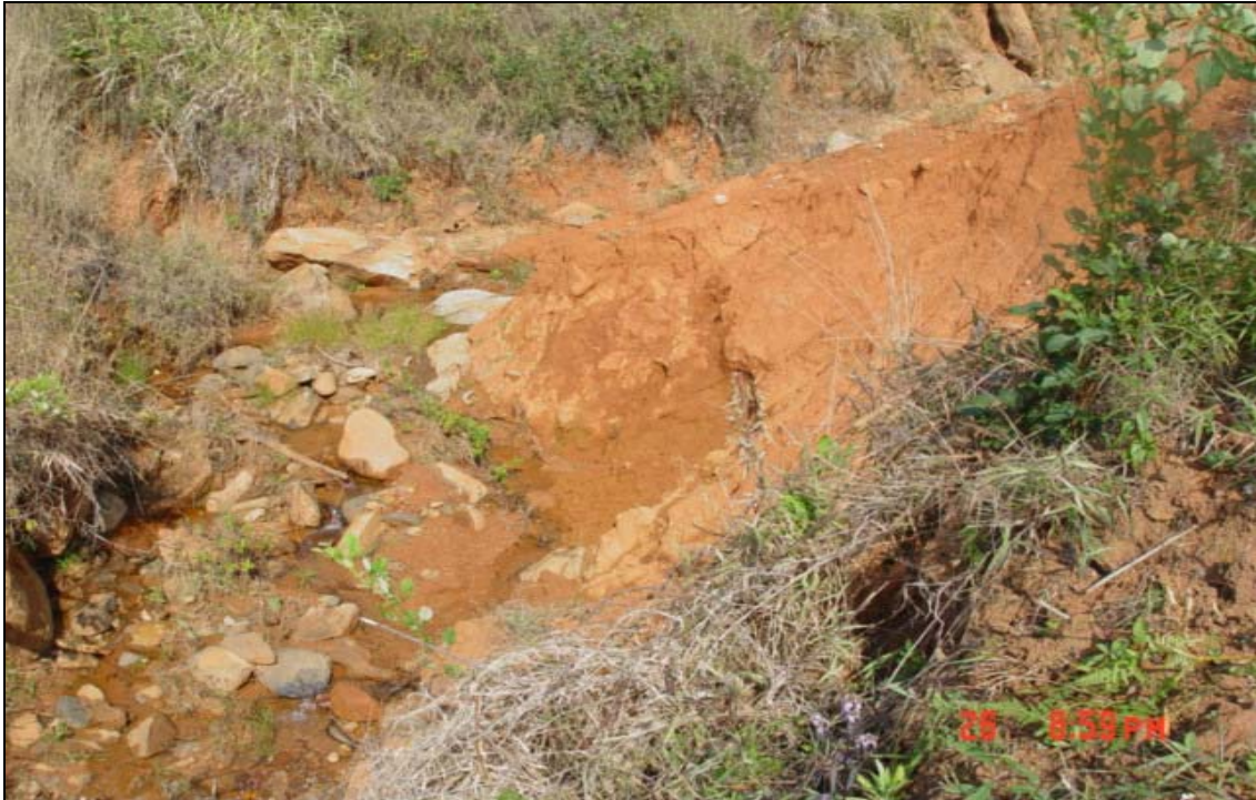
Figure 6.12: Position where landslide debris dammed the Lutowo River which resulted in the flooding of Mzinga River. Debris remains can be seen at the site (26.08.06).
