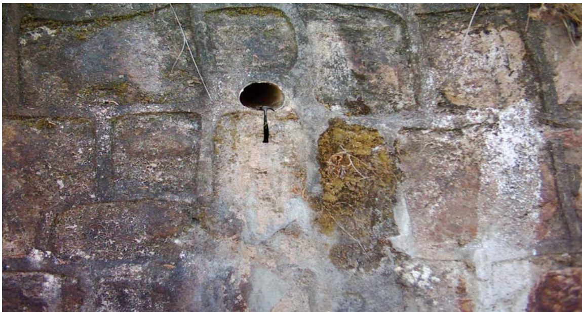
Figure 9.2: Concrete stone embankments constructed to stabilise landslide prone slopes at Overtoun in Northern Malawi. Note the plastic tubing to prevent the build up of water table (11.08.01).
