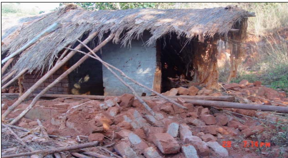
Figure 8.2: Remains of the abandoned settlement at Mwachumba Village at Ntchenachena after the 2003 landslides. Note the material of material used which increased the risk of failure (29.08.06).
