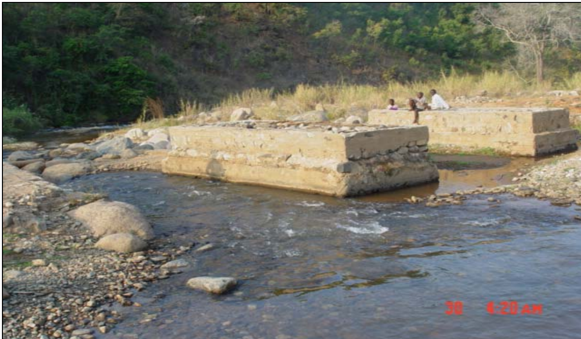
Figure 6.8: The remains of the Phoka Bridge at the confluence of the Mzinga and the North Rumphi Rivers after the 2003 landslides in the Ntchenachena Area (30.08.06).
