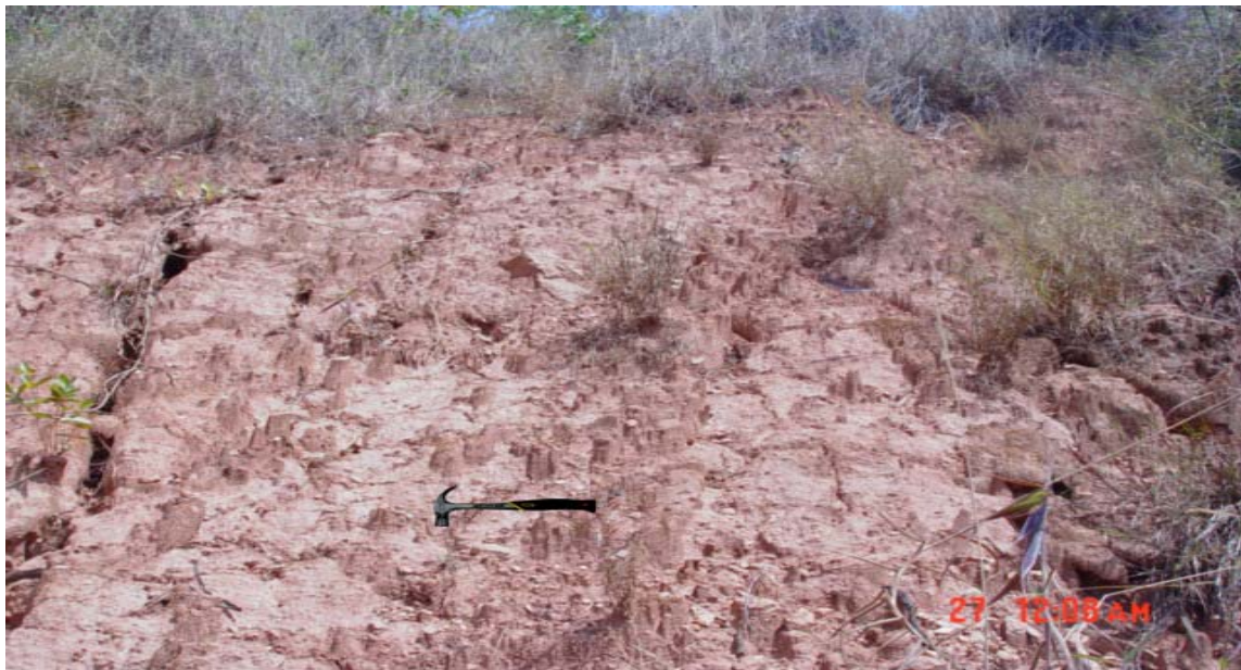
Figure 7.8: Soils which liquefied and dried are common in the all study areas. The photo represents liquefaction at the Lutowo unit of the Ntchenachena Area (27.08.06).
