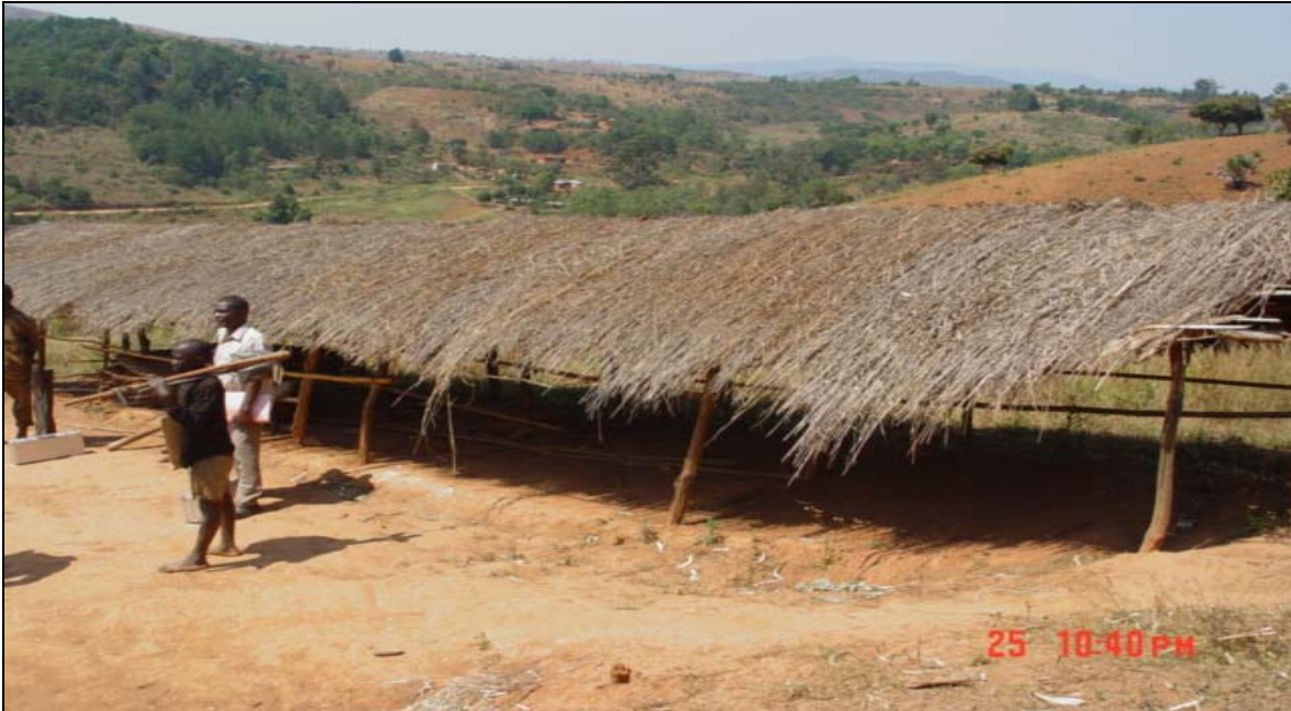
Figure 2.10: Tobacco curing shed in the Ntchenachena Area, contributing to deforestation. Note that the location of the Shed is on a remodeled slope affecting the balance of forces operating in slope (25.08.06).
