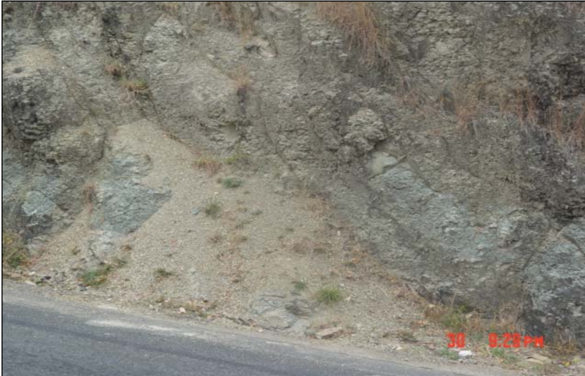
Figure 7.16: Highly weathered Chiweta beds dipping along the main road to Karonga. Note the creeping of weathered colluvium at the base of the cliff (30.08.06).
