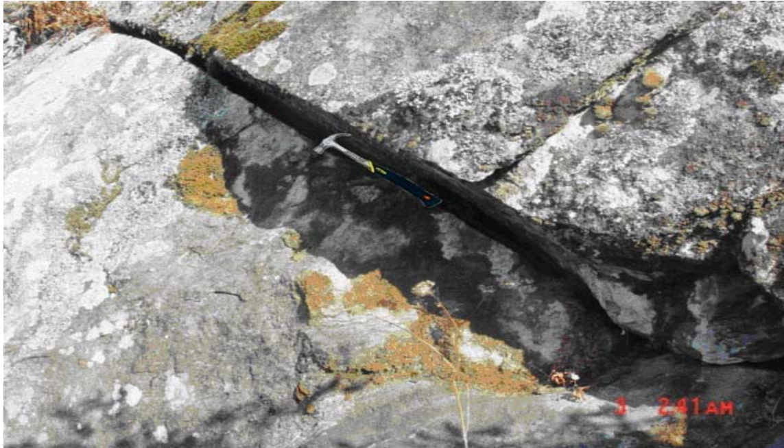
Figure 7.9: Structural rock weaknesses through which water penetrated, causing high cleft pressure and land sliding at the Mvai Study Area (3.09.06).
