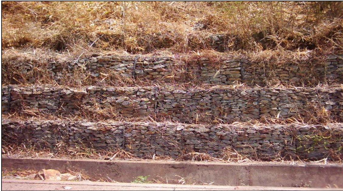
Figure 9.1: Stone embankments, using wire mesh, constructed to stabilise Nyankhowa slopes in Northern Malawi. Similar structures can be used to stabilise the Chiweta beds (11.08.01).
