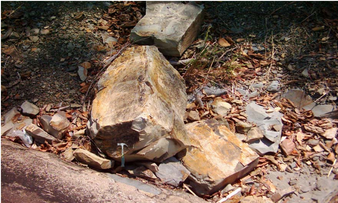
Figure 6.9: Rock falls along the M1 Road to Karonga, typical of the Chiweta beds. These have been a major cause of accidents (29.08.06).
