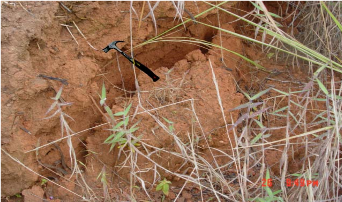
Figure 7.1: Soil cracking and deformation; an indication of instability, common in the Ntchenachena and the Livilivi Areas (Photo taken at Ntchenachena 26.08.06).
