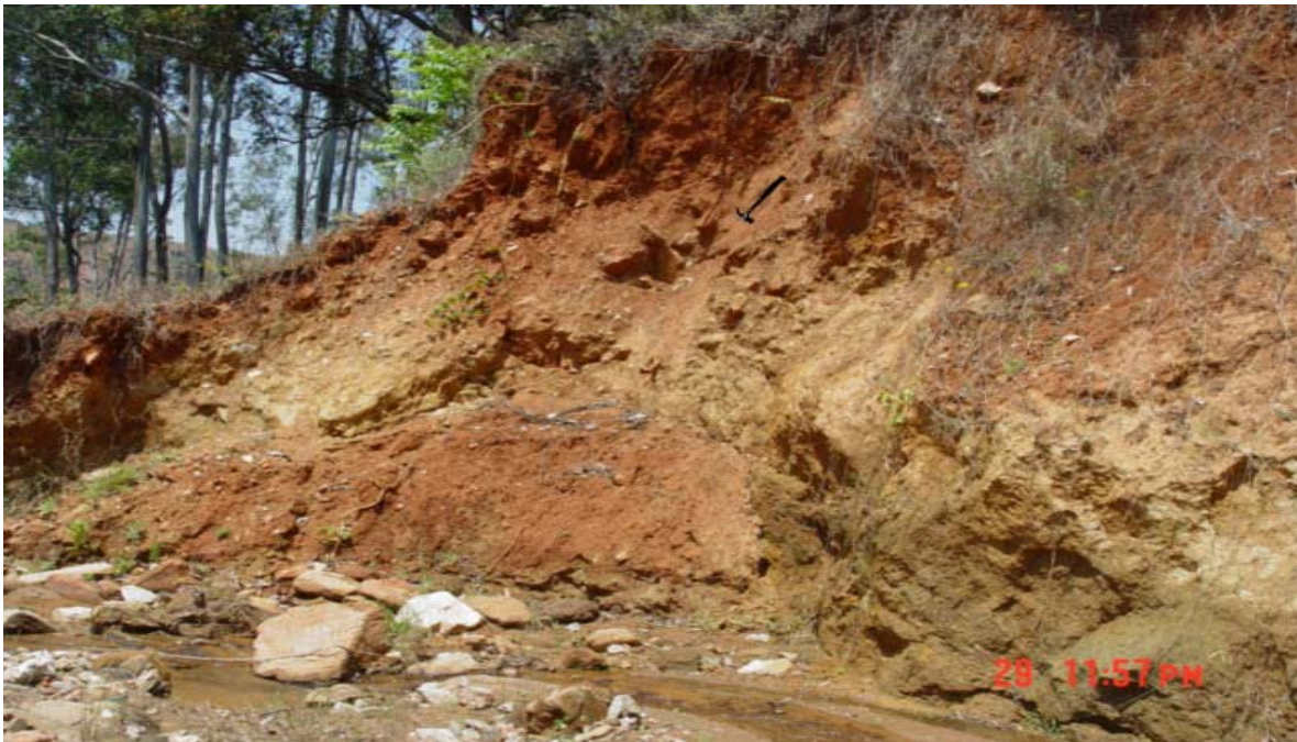
Figure 6.13: Bank collapse caused by landslides, common at all Study Areas and contributing to siltation of rivers. This is an example from the Livilivi Catchment (28.08.06).
