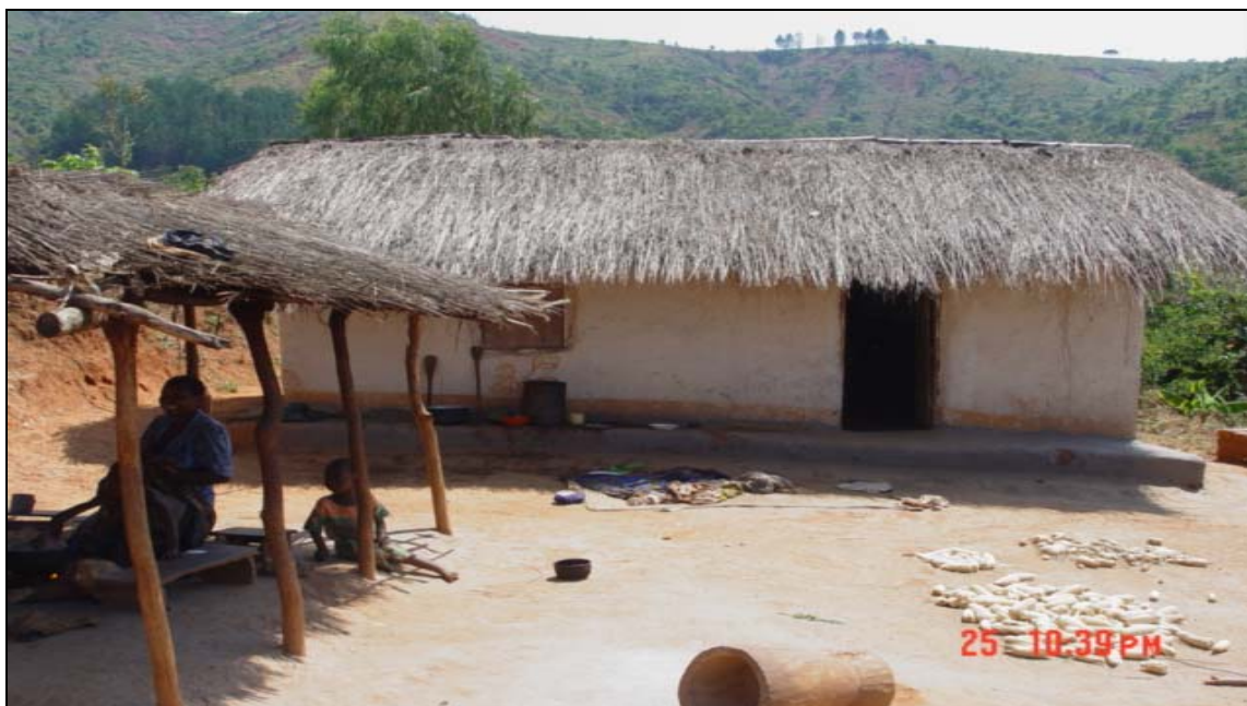
Figure 8.1: Traditional houses common in rural areas of Malawi. This house is built on an excavated slope in the Ntchenachena area (25.08.06).
