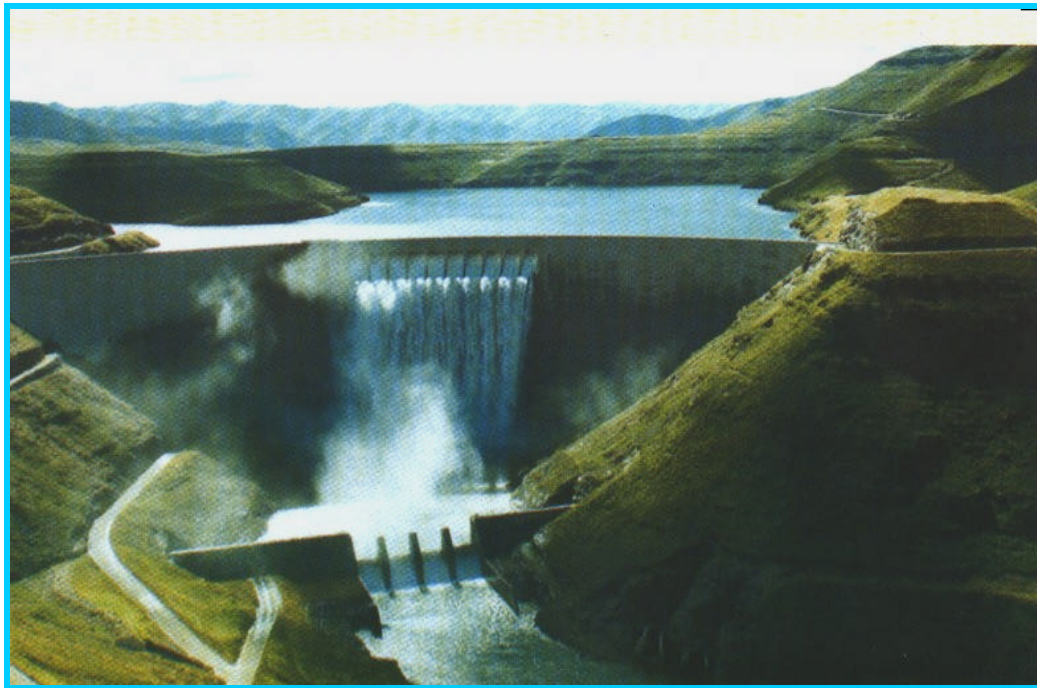
Fig. 4.12b: Katse Dam downstream flood (LHDA, 2002g).
