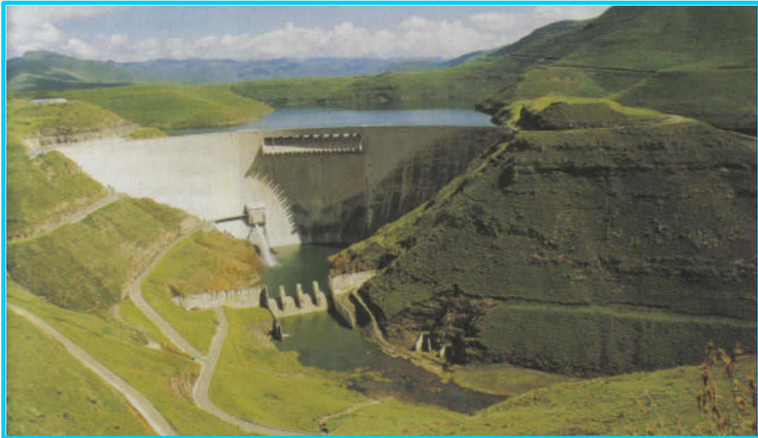
Fig. 1.5: Phase 1A Katse Dam Wall. The highest dam wall in Africa (LHDA, 2000b).
