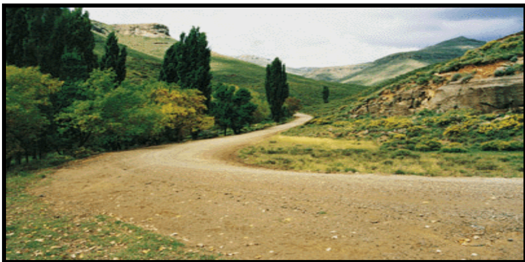
Fig. 3.9: LHWP rural access gravel road (TCTA, 2003b)
