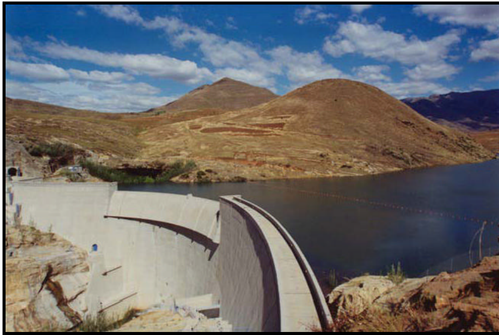
Fig. 1.6: Phase 1A Muela Hydro-power Dam (72MW) (LHDA, 2005)
