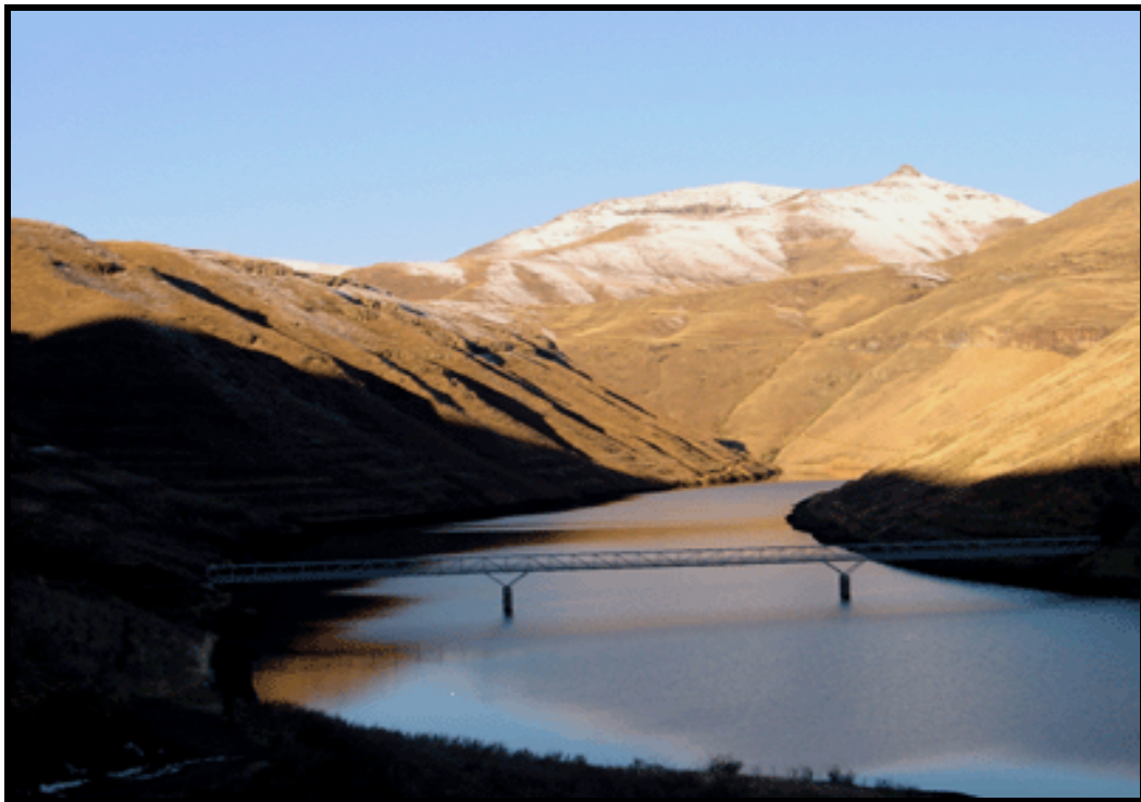
Fig. 3.12: Ha Katse: Bokong Foot Bridge (TCTA, 2004a)
