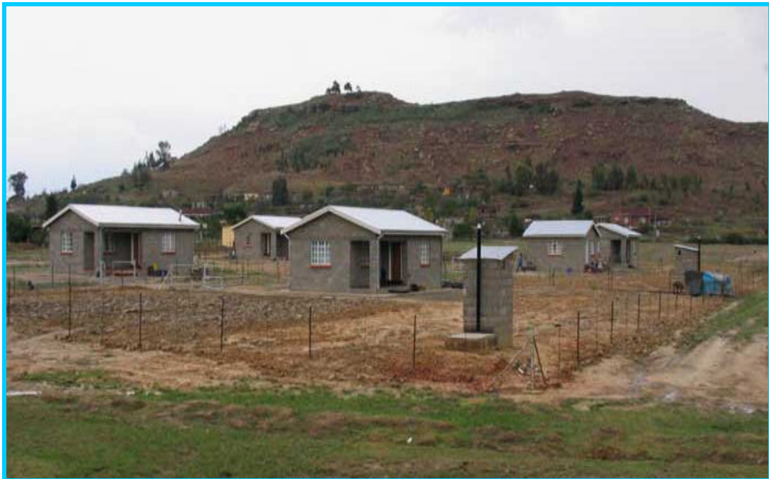
Fig. 4.7: Ha Makhalanyane: Fenced resettlement houses for affected communities (LHDA-SAICE, 2003b)
