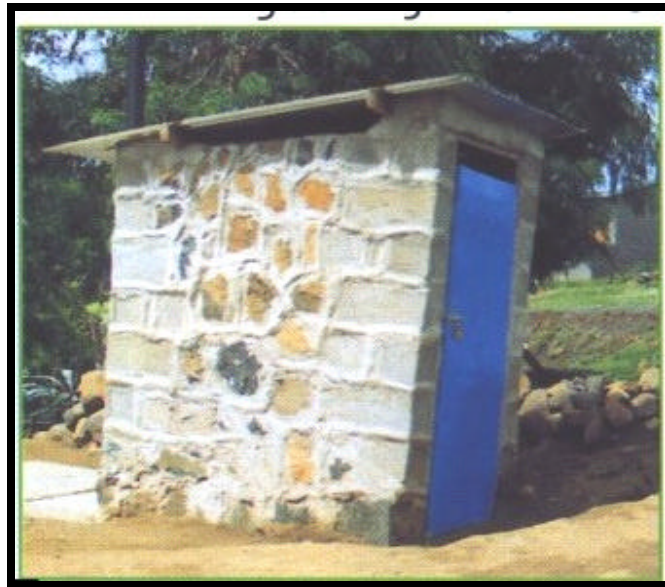
Fig. 3.15: Muela: Typical VIP toilet, a convenience near the house (LHDA, 2002d)
