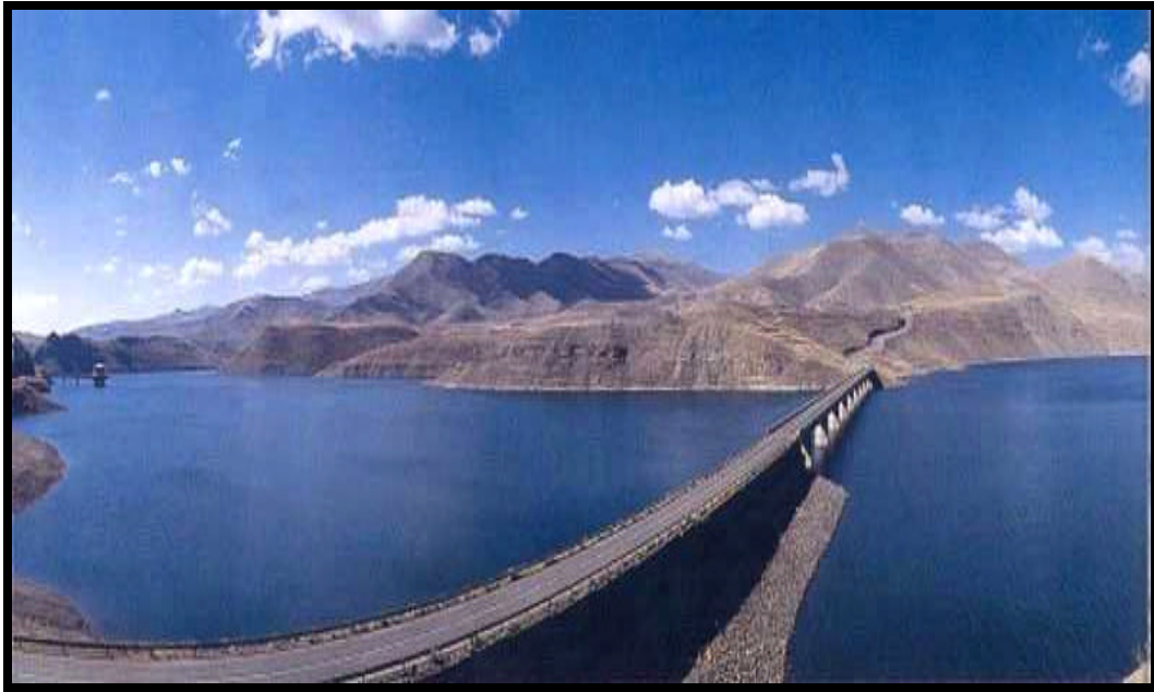
Fig. 3.11: Malibamatso Bridge, the tallest in Africa, crosses all traffic over Ha Katse Reservoir (LHDA –TCTA, 2001)
