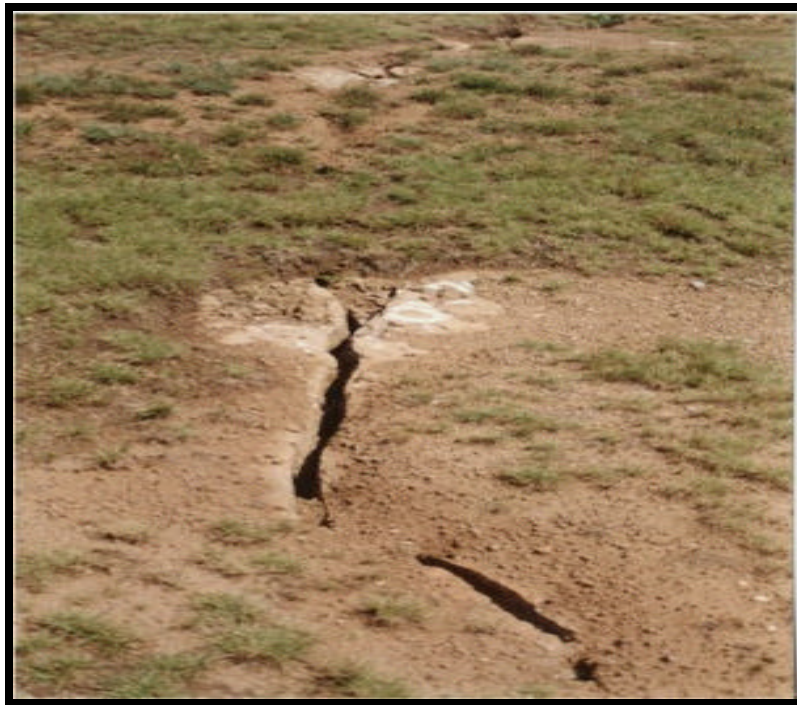
Fig. 4.14: Reservoir induced seismicity caused some unusual ground cracks in Ha Katse area (LHDA-SAICE, 2003b).
