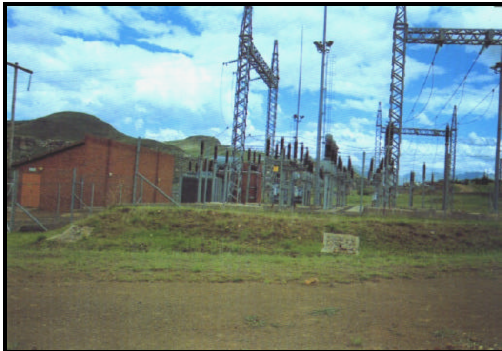
Fig. 4.15: Khukhune Electric Power Substation ensuring electricity to urban areas (LHDA, 2002d).
