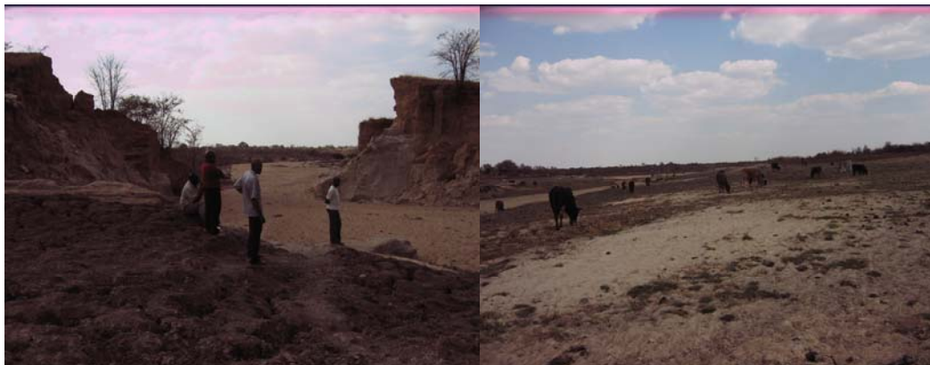
Figure 10: Shagari dam wall destroyed by excessive rains (2009 Survey)
