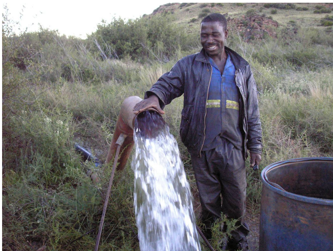
Figure 7-3: Fickson from AB Pumps at riser pipe yielding 25 \ell/s from EC-Q14-1655 during its constant discharge test
