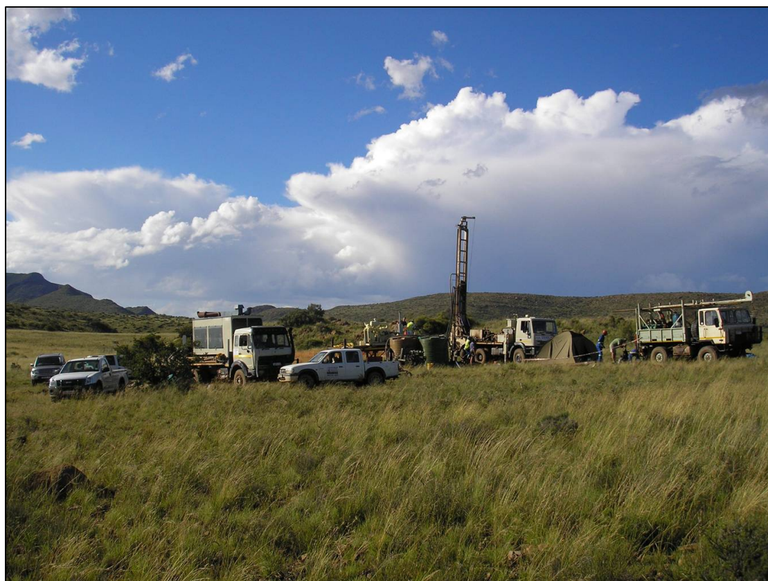
Figure 6-9: Water Hammer operations at EC-Q14-1636
