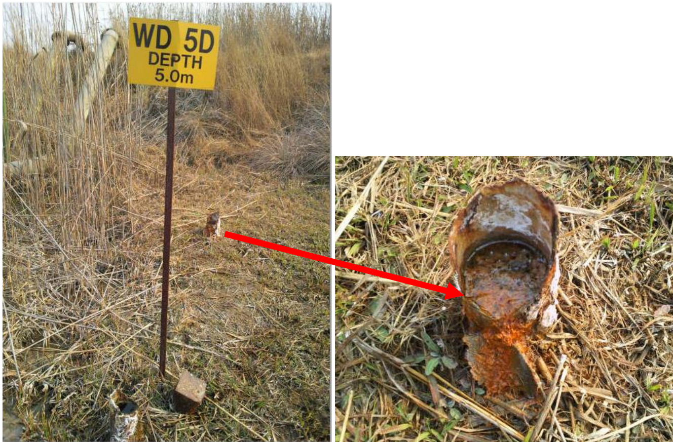
Figure 3-22: Boreholes in vicinity (approx. <10m) of the return water dam corroded /deteriorated due to acidic water by SO 4
