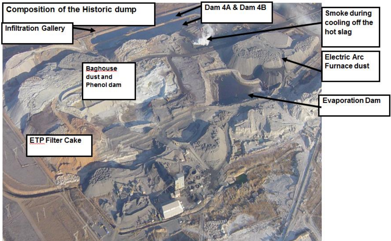
Figure 3-12: Aerial photo of the historical site dump of the study area
