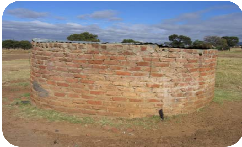
Illustration 4.1: A dam in need of repairs
