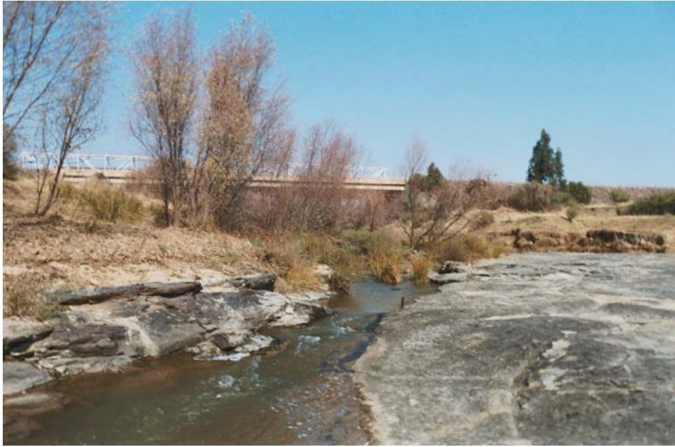
Plate 5.8: Significant changes to the channel below a weir and bridge (MR 3) prevented by lack of sediment inputs
