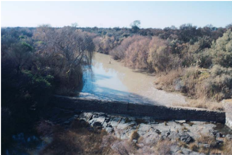
Plate 5.7: Sediment transport restricted by a structure
