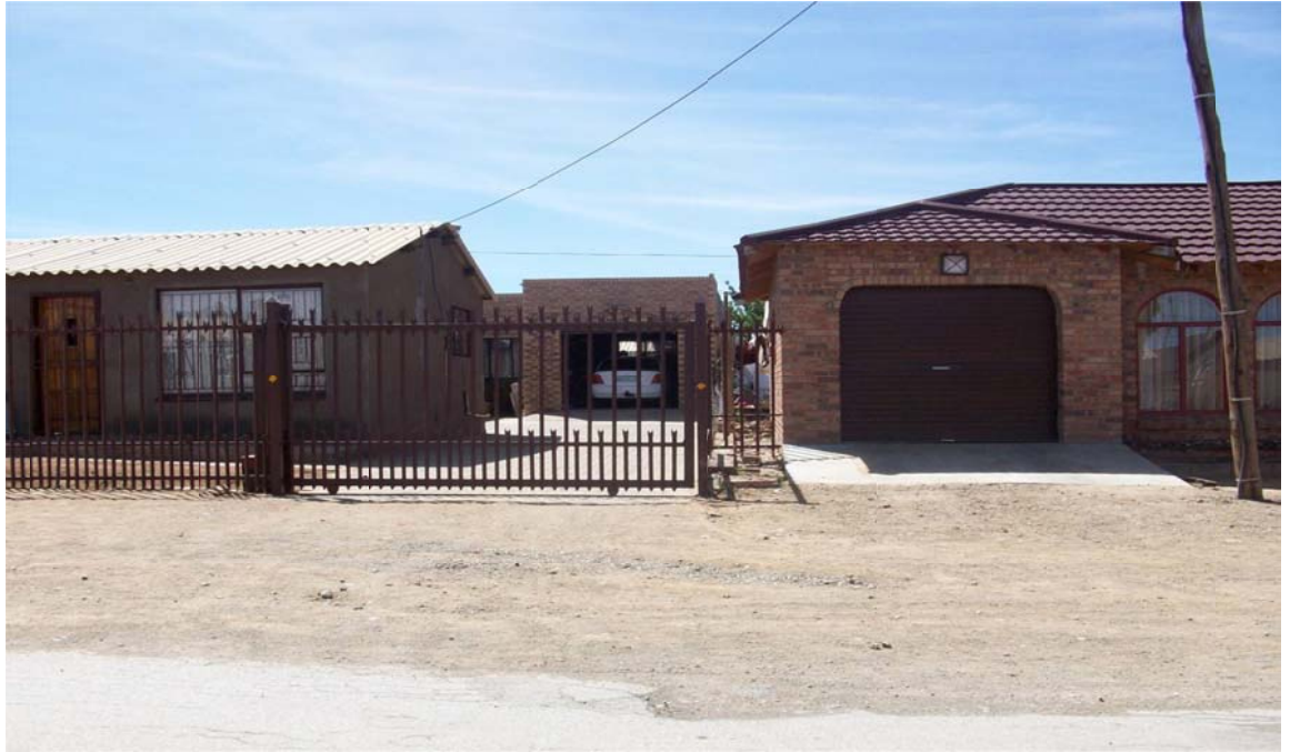
Plate 11: The picture depicts the common form of transformation (detached backrooms).
