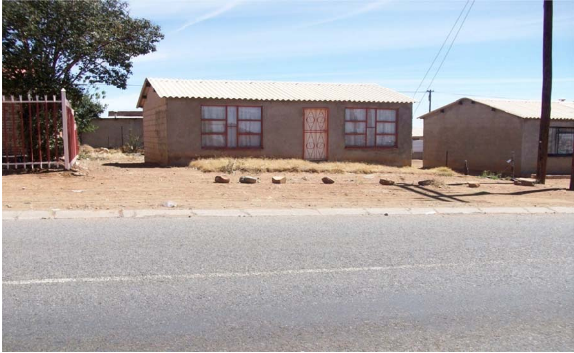
Plate 6: A rental prototype with improved windows and burglar door, but without fencing
