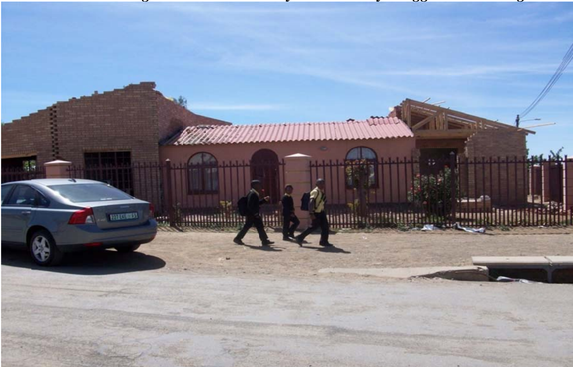
Plate 3: The original rental unit slowly swallowed by a bigger house being built.
