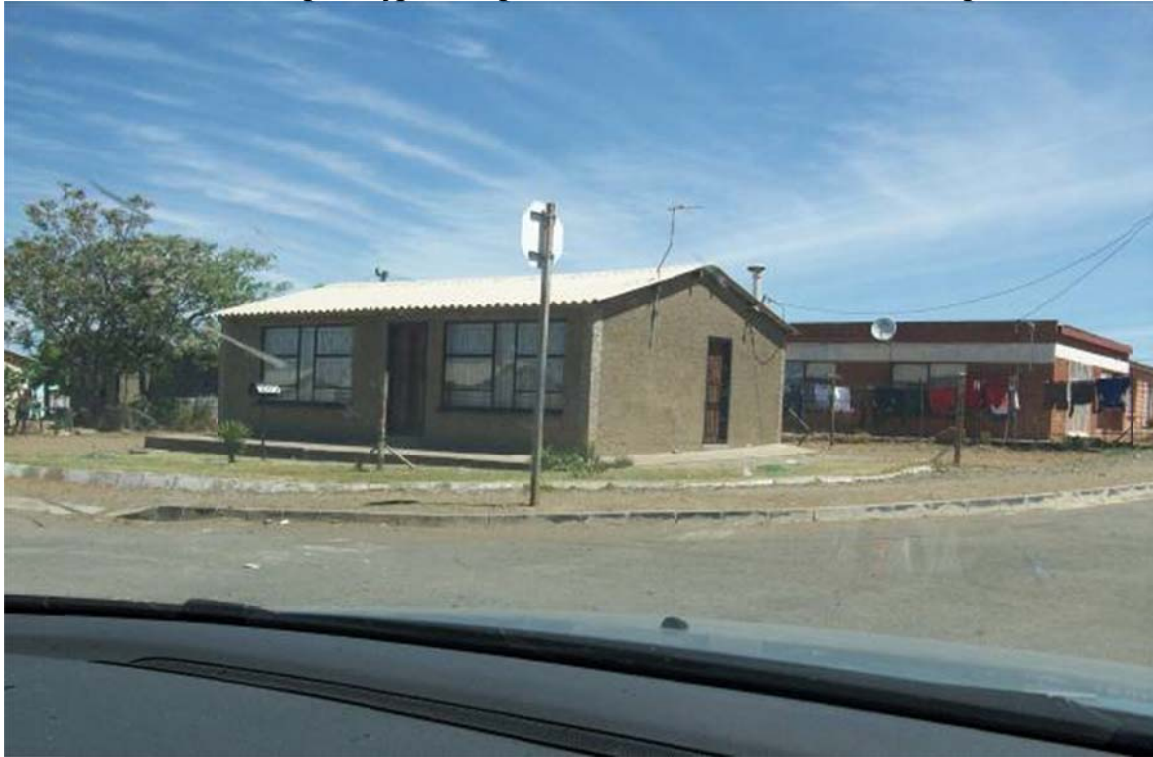
Plate 8: A rental prototype with plastered exterior walls and a “stoep”
