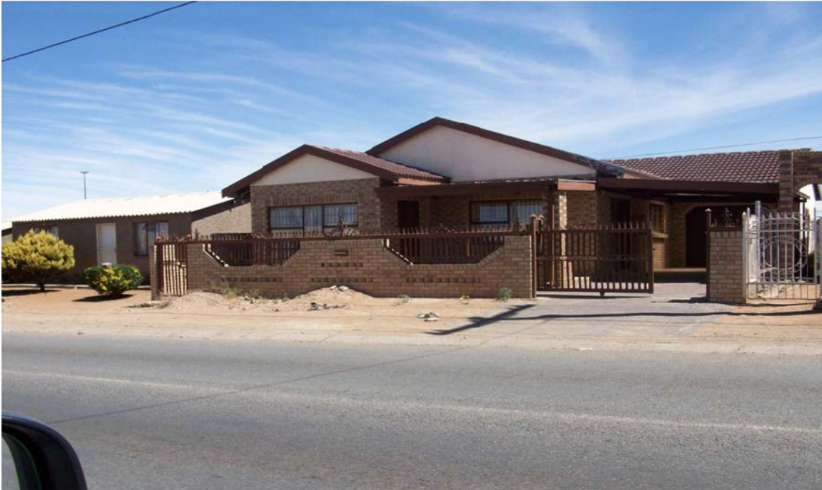
Plate 2: A core house has been demolished or subsumed into a new and bigger house
