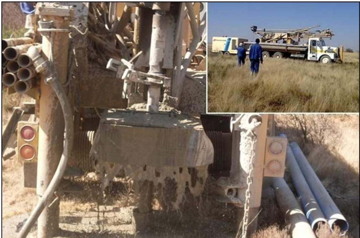
Figure 4-8: Cable tool method and cable tool rig (insert) used for drilling at the study site.
