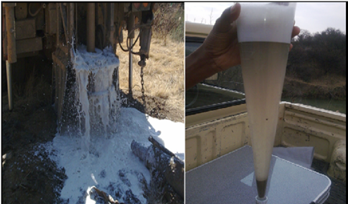
Figure 3-5: Borehole backwashing development with the aid of the rotafoam and the settleable solids test using Imhoff cone.
