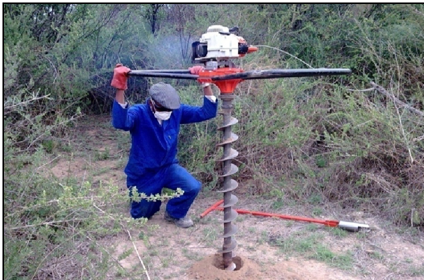
Figure 4-3: Auguring of the holes on which infiltration test was executed.
