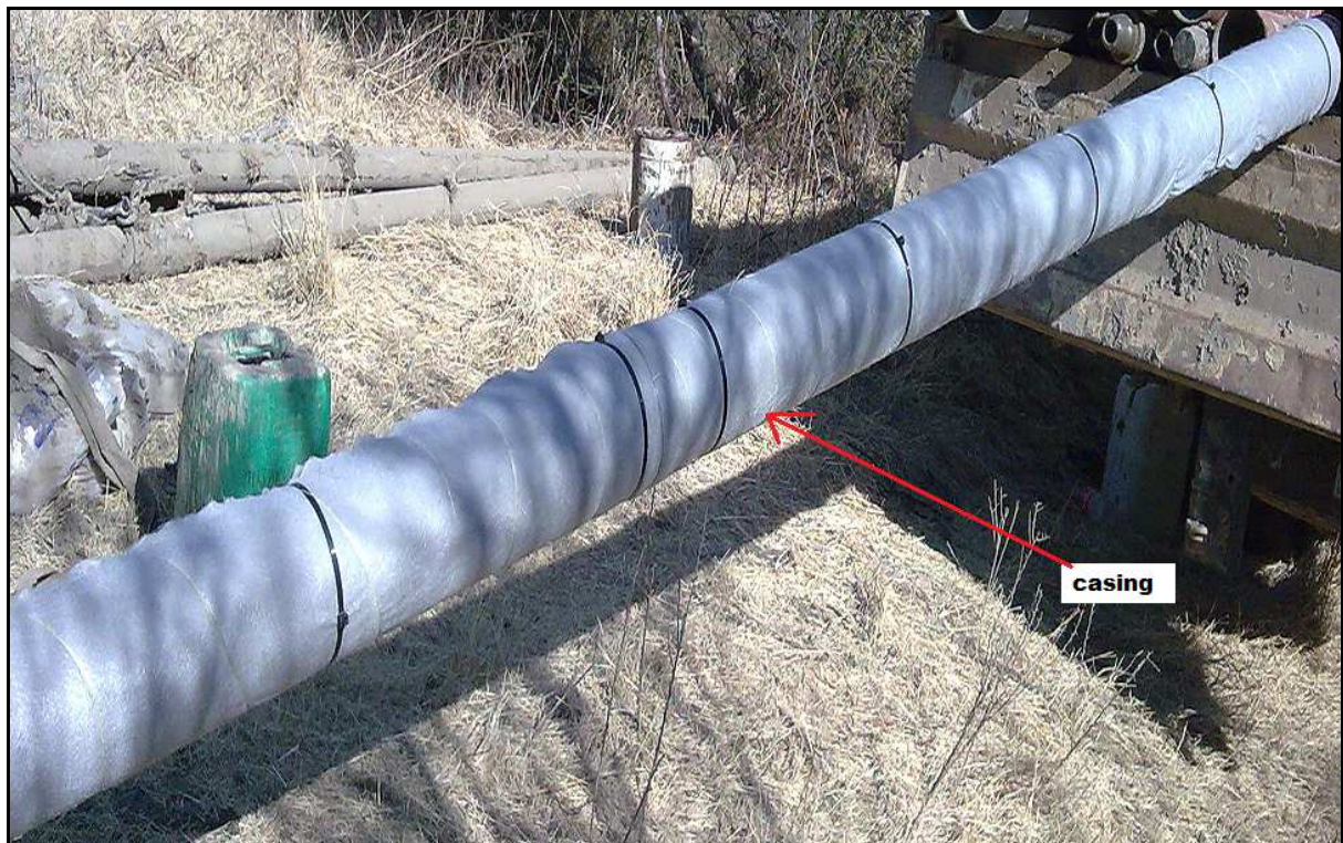
Figure 3-3: Inside casing wrapped with a fine mesh (bedim).
