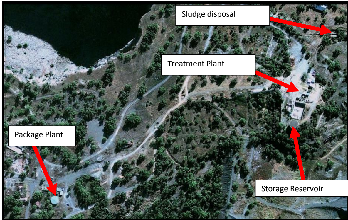
Figure 5-2: Picture showing location of plants and sludge disposal site
