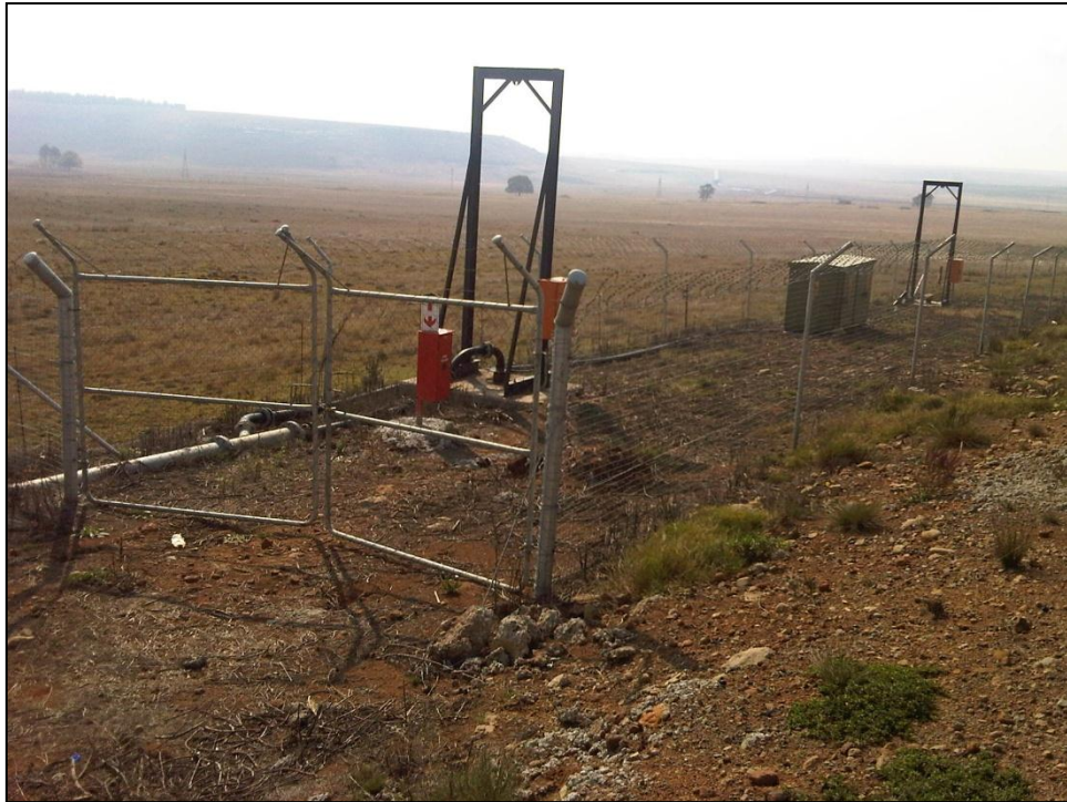
Figure 7-43: Photograph of the extraction wells pumping water from Usutu South to Mooiplaats Colliery.
