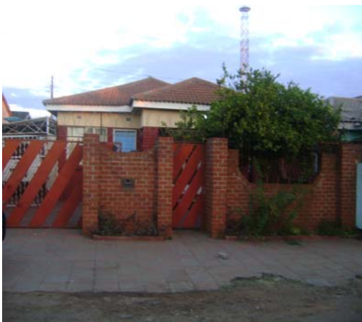
Self constructed cooperative houses in Dzivarasekwa
