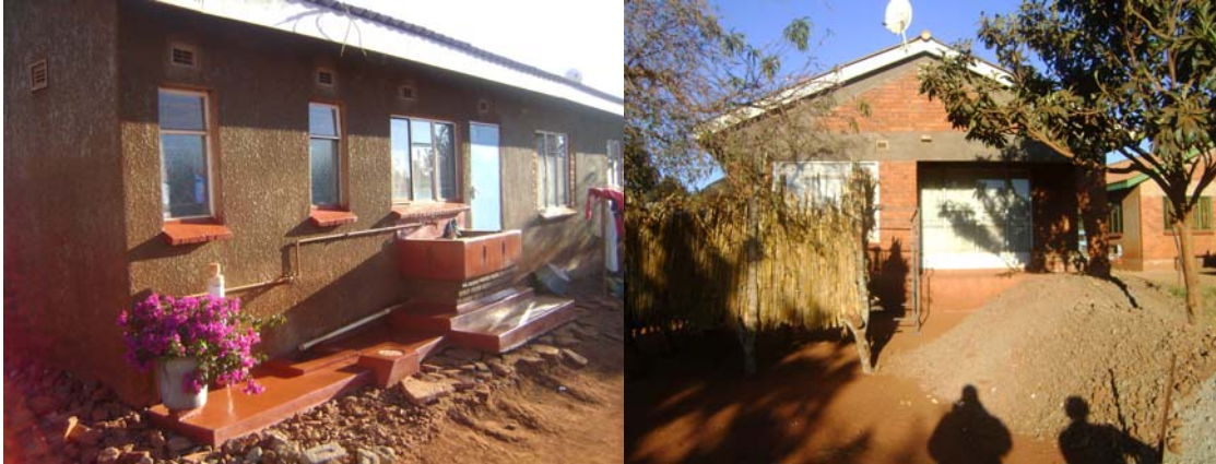
A transformed cooperative house built by a former squatter in Hatcliff.
