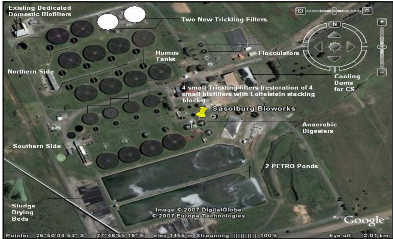
Figure 13: SCI sewage treatment plant (Reddy, 2008).
